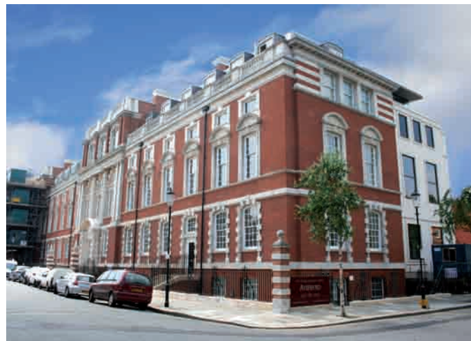
The retained facade fronting Manresa Road, with the new garden facade visible to the right
