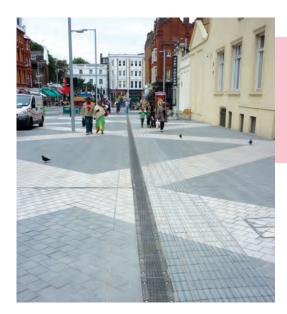
Black cast iron drainage channel covers run along each side of Exhibition Road, about four metres out from the respective building lines. Alongside the drainage channels strips of corduroy tactile warn blind and partially sighted people that they are moving into or out of vehicle free areas.
