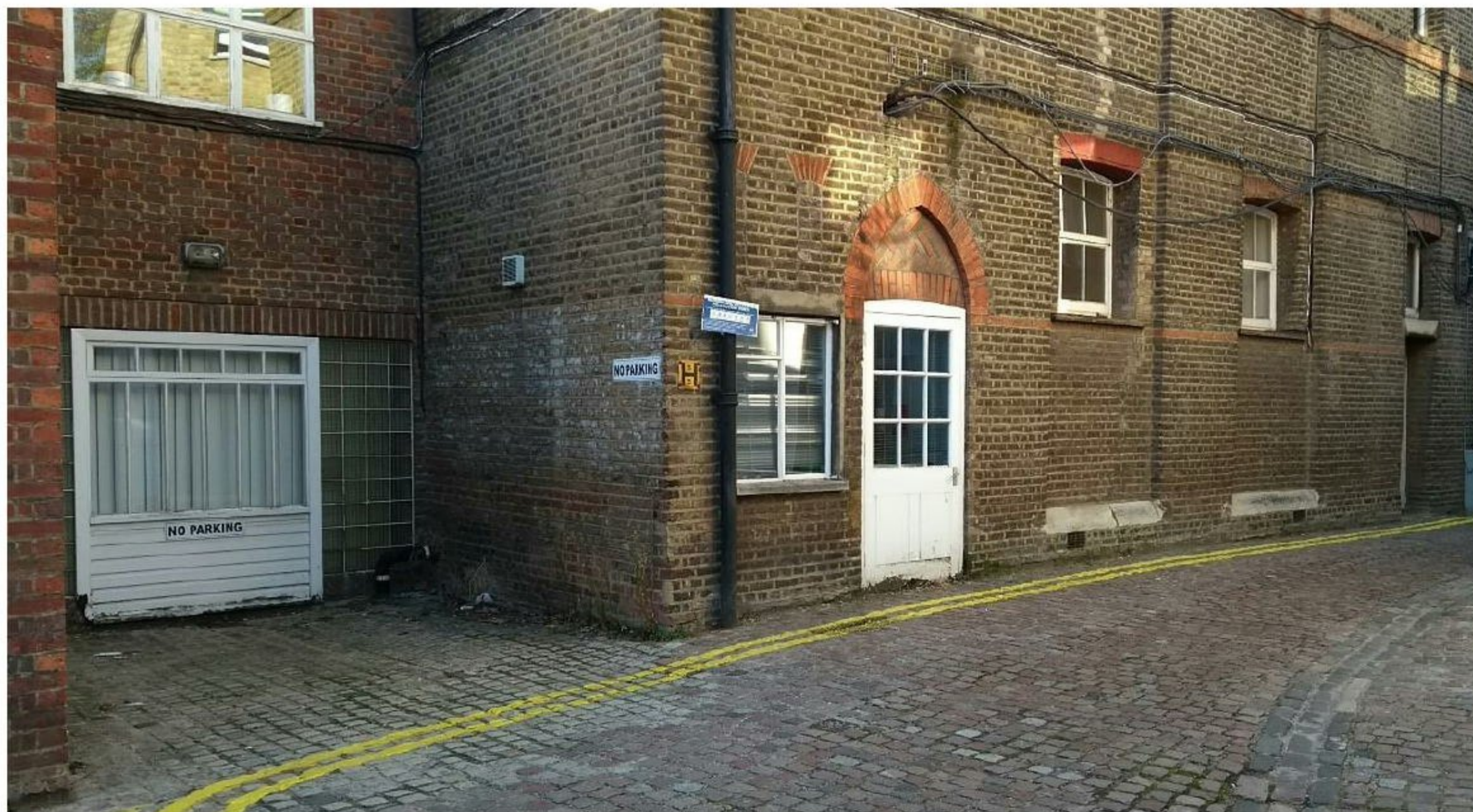
Plate 6: Turning area outside No 10 South End
