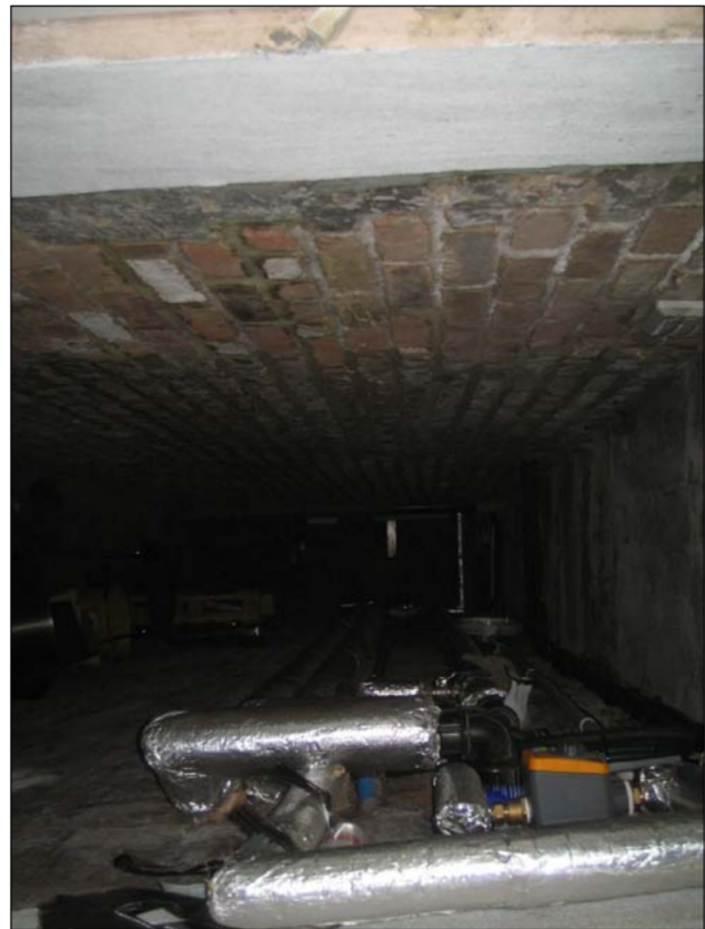
VIEW INTO FRONT LIGHTWELL
