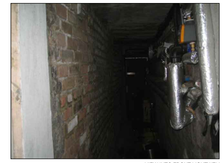
VIEW INTO FRONT LIGHTWELL
