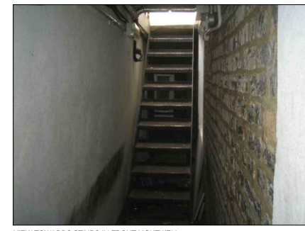
VIEW TOWARDS STAIRS IN FRONT LIGHTWELL
