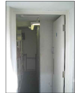
VIEW INTO EXISTING COVERED LIGHTWELL
