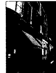
EXISTING COVERED LIGHTWELL
