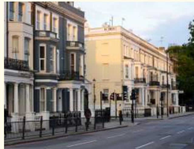
3. Warwick Road looking south to Penywern Road
