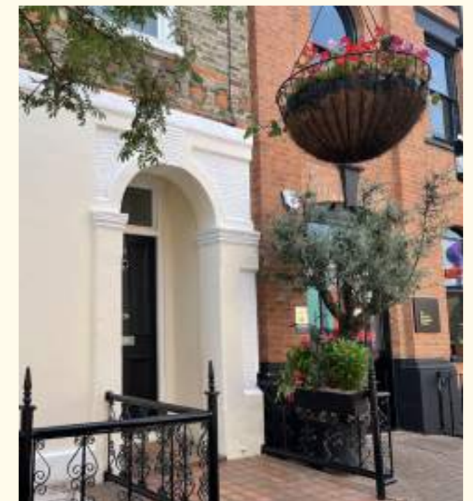
6. View of the western terraced houses on Empress Place
