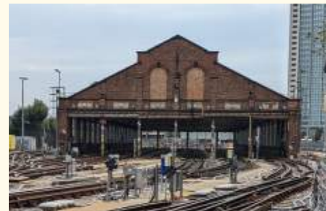
4. View of the northern gable of the Train Shed
