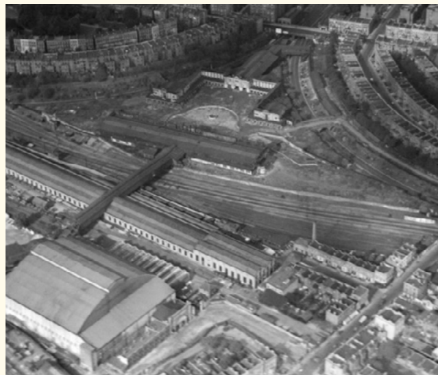
Aerial view, 1928. The Train Shed can be seen extending the length of the Site to Empress Place. © Historic England
