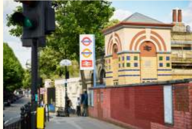
1. Entrance to West Brompton station
