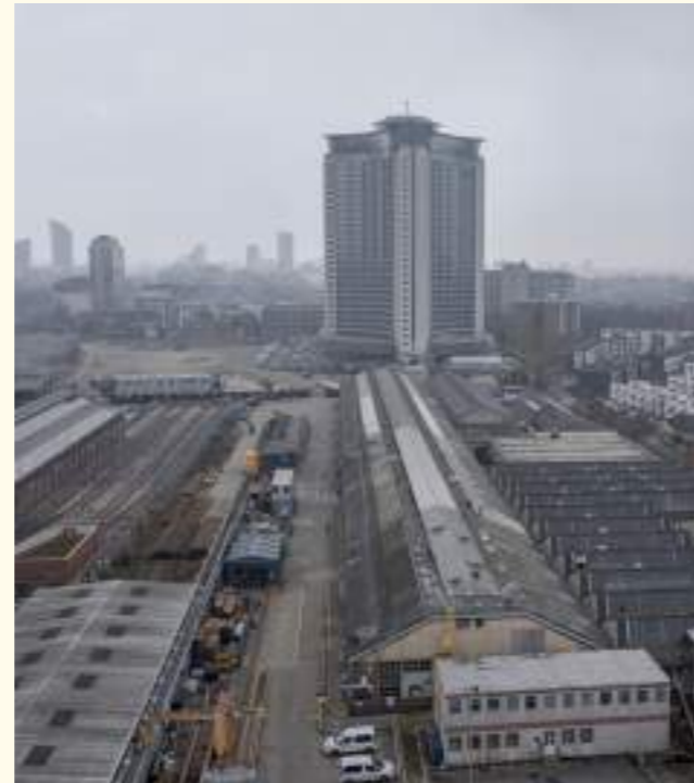
1. View looking south over the Lillie Bridge Depot
