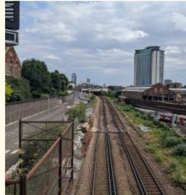
4. View looking south along the Northern Access Road and West London Railway Line
