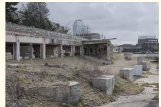
8. Remaining concourse structure adjacent to Eardley Crescent
