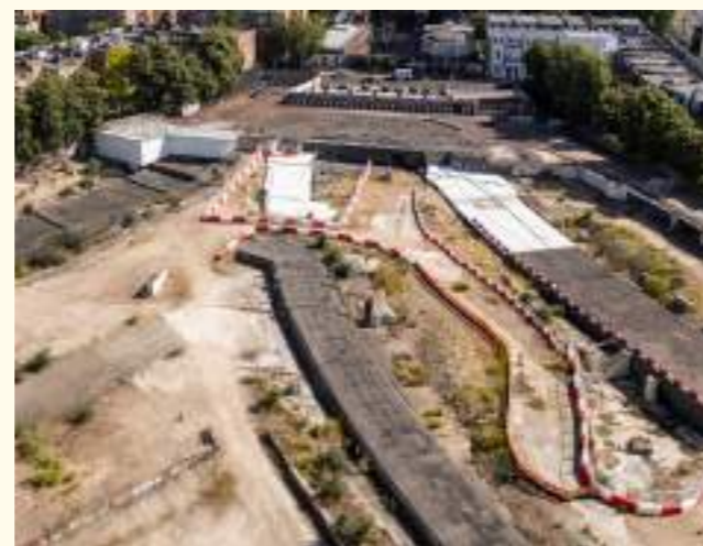
3. View looking east showing the tops of the District Line tunnels
