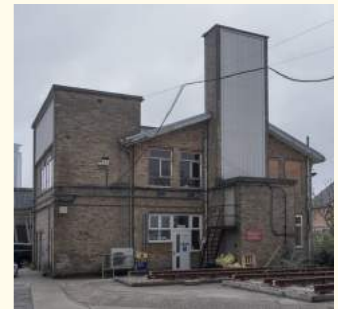
7. Existing TfL operational building
