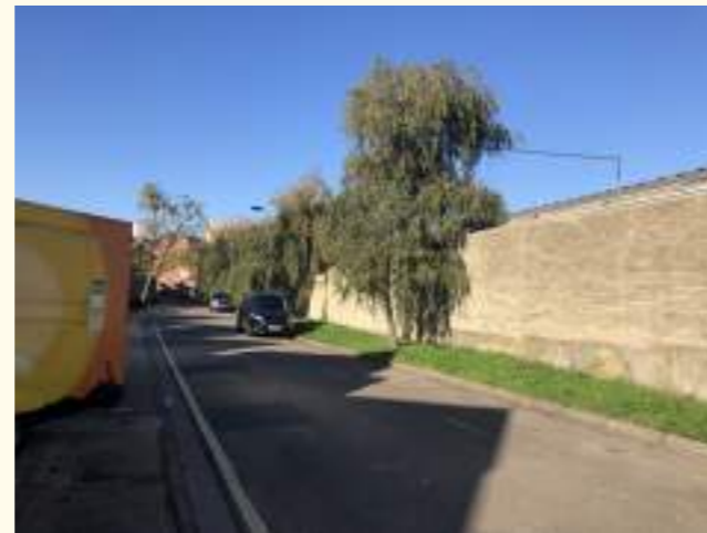
2. The boundary wall between West Kensington and Gibbs Green Estates, and the Site
