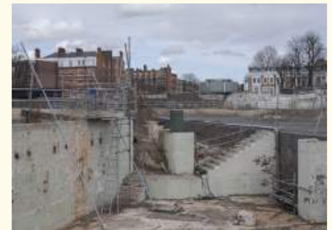
7. Remaining structures adjacent to District Line tunnel
