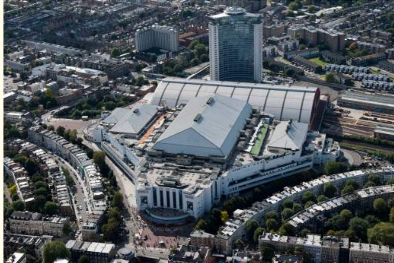
Aerial view of the Earls Court Exhibition Centres before demolition
