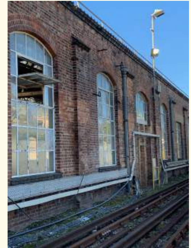
6. View of the western facade of the Train Shed
