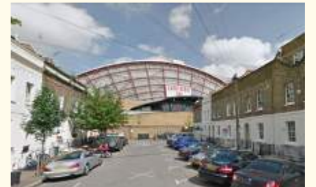
View of EC2 from Empress Place ©Google Streetview
