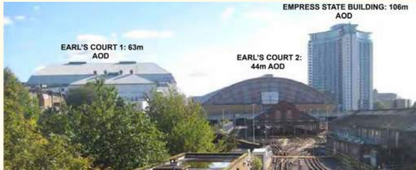
View from West Cromwell Road of the former Exhibition Centres, with approximate heights Above Ordnance Datum (AOD)
