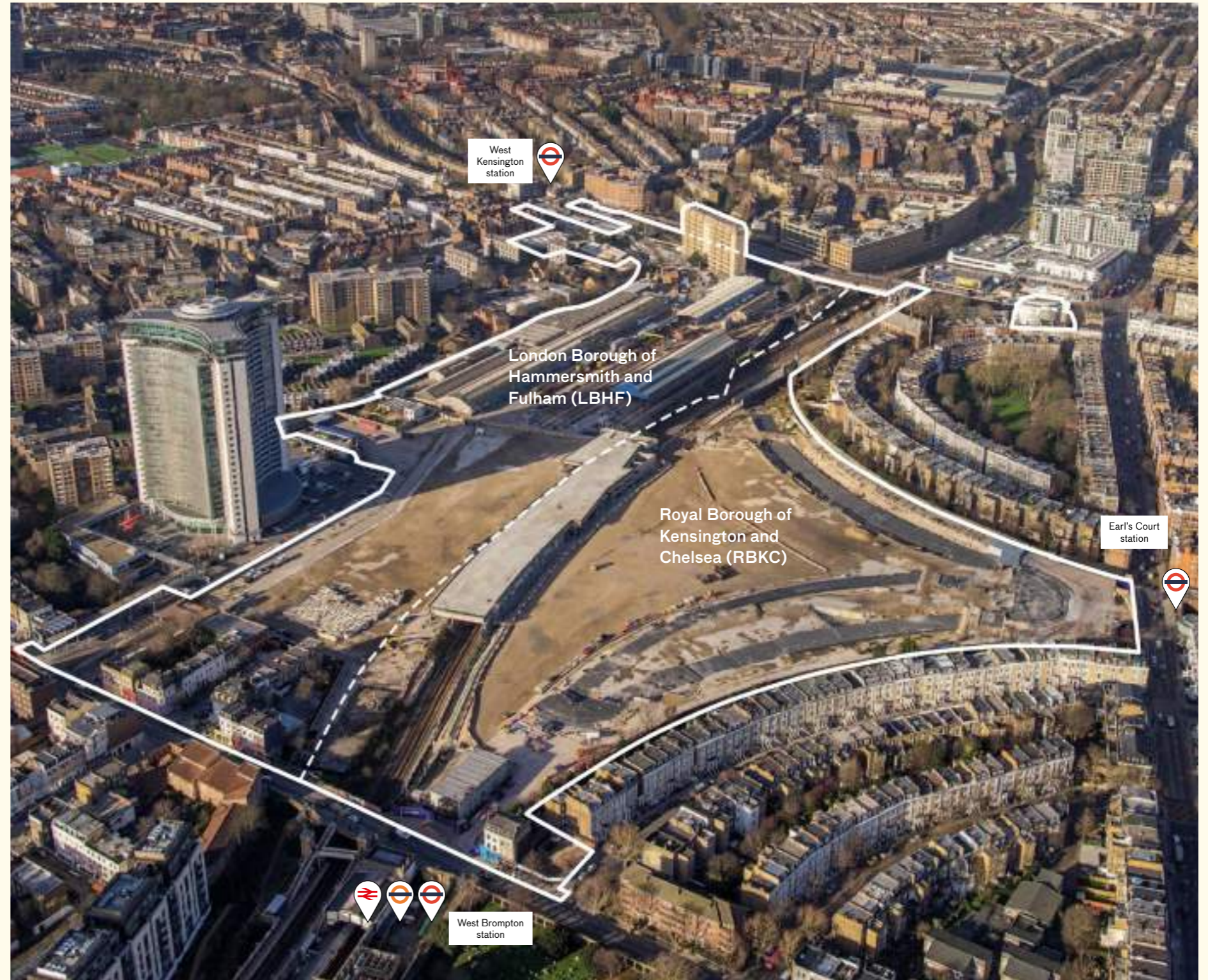
Aerial view of the Earls Court Site
