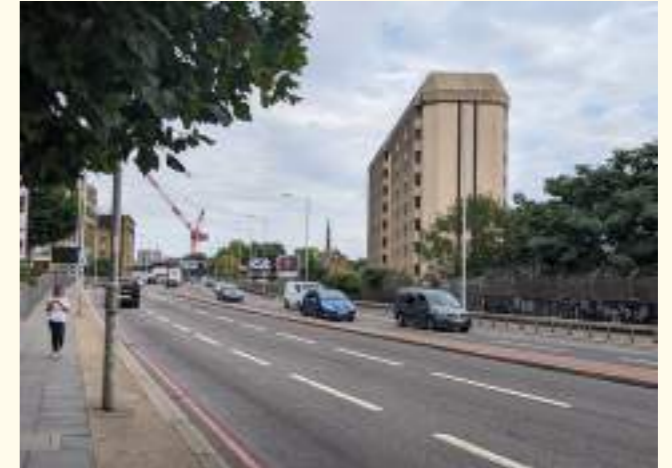
1. West Cromwell Road looking east
