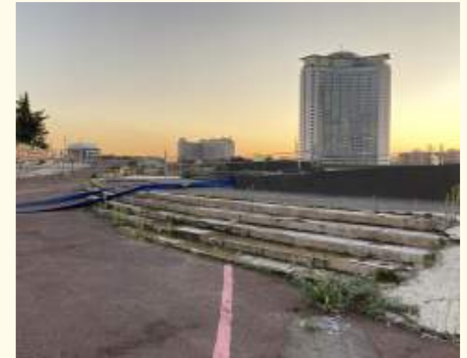
6. Remaining steps of former Exhibition Centres entrance
