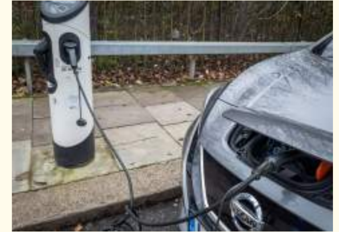
Electric vehicle charging point
