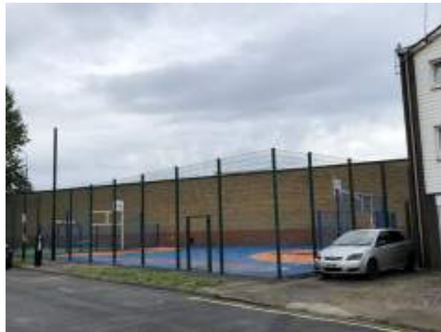
Existing triangular sports area and brick wall
