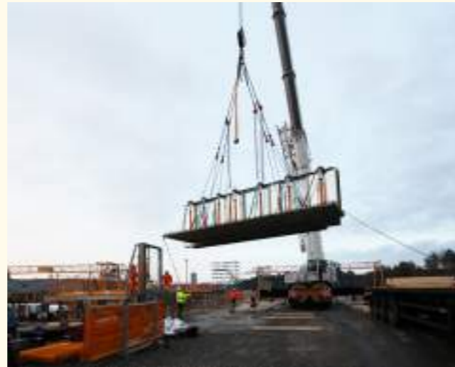
MMC: Prefabricated building elements can reduce time spent on-site
