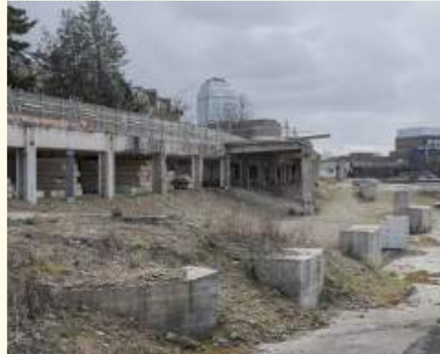
Concourse structures and foundation have been assessed.
