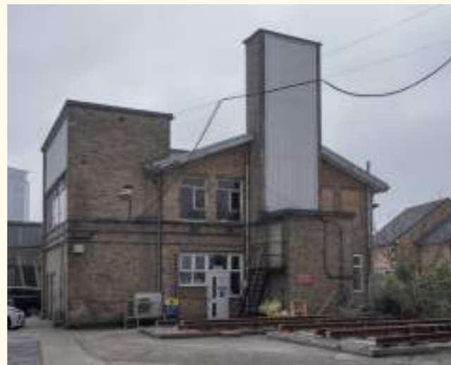
All existing buildings have been assessed against the requirements for the Site, alongside an initial qualitative and quantitative assessment of their materials.
