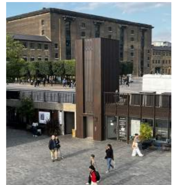
Example of integration of lift access to assist with the level change
