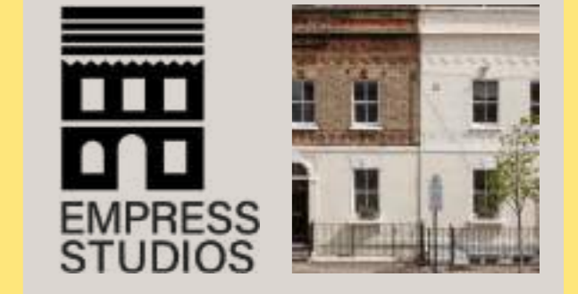
The transformation of Empress Place terraces into Empress Studios, a collection of 46 artist studios
