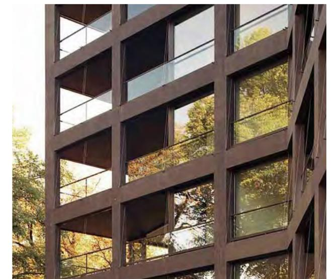
Fig 4.29: Building 2.6 - Example of linear/recessed balconies
