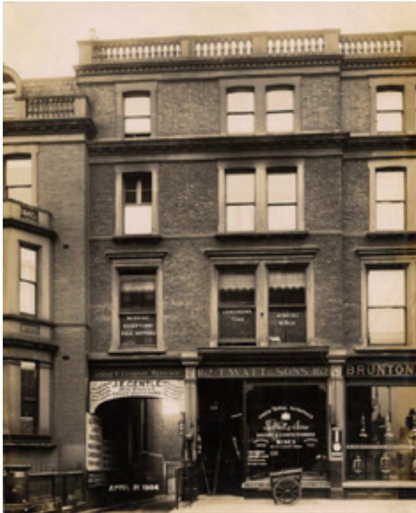
240-242 Earl's Court Rd & Old Manor Yard
