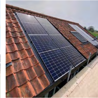
PV installation on a roof (house) as tile replacement
