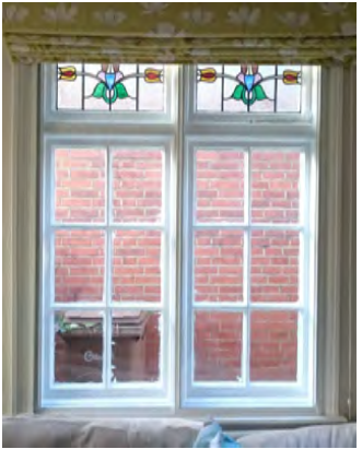
Secondary glazing in front of historic stained glass
