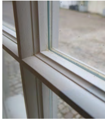
Evacuated glass sash windows within a conservation area
