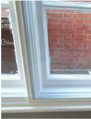
Secondary glazing in front of historic stained glass
