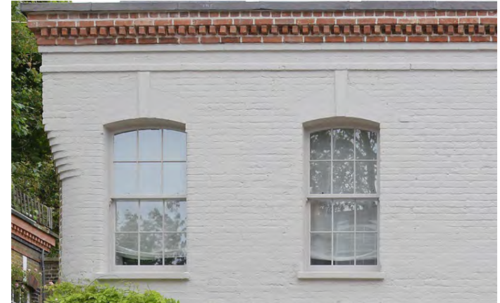
Exterior view of evacuated glazed sash windows in combination with internal wall insulation, in a conservation area in RBKC .
