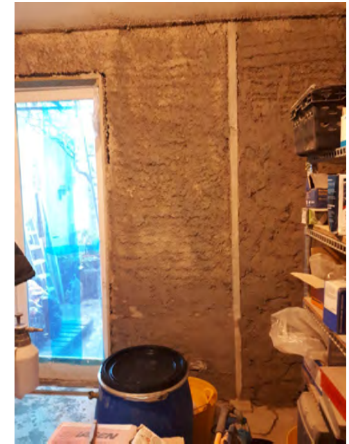
Initial coats of lime/cork plaster being sprayed onto a masonry wall
