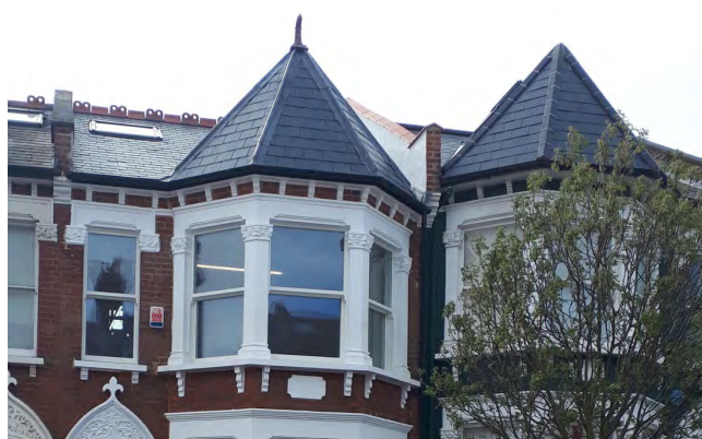
Triple glazed mock sash window
