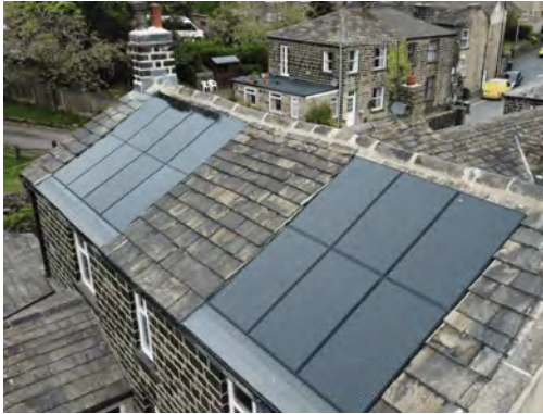
PV installation on a roof (house) as tile replacement
