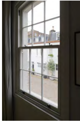
Evacuated glass sash windows within a conservation area
