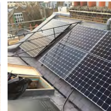
PV installation on a roof (house) over the tiles
