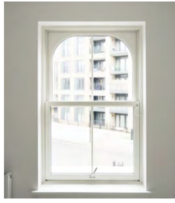
Double glazed sash window within a conservation area
