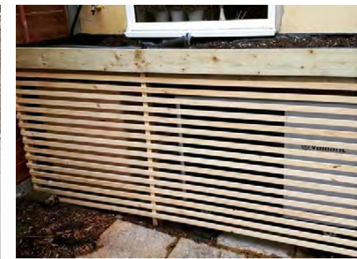
Heat pump under a window and behind enclosure
