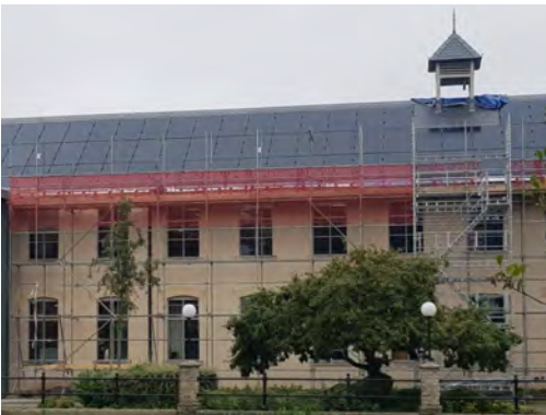
PV installation (rear elevation) over the tiles
