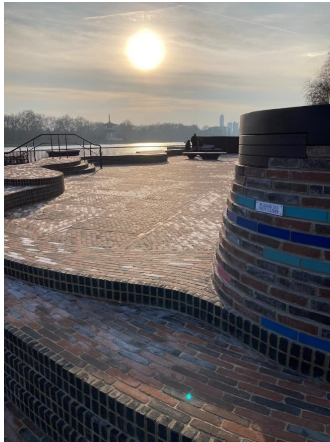
New public realm at Chelsea Embankment Tideway Tunnel site
