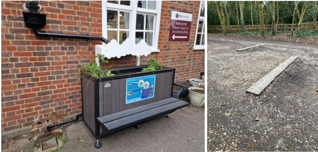
SuDS Planter in Avondale Primary School (left), pathway NFM in Holland Park (centre)
