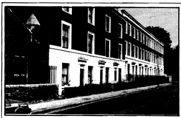
Caversham Street – north side
