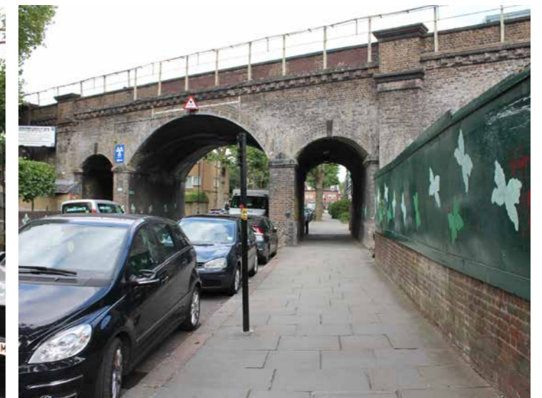
4. Pavement view of the railway viaduct and arches
