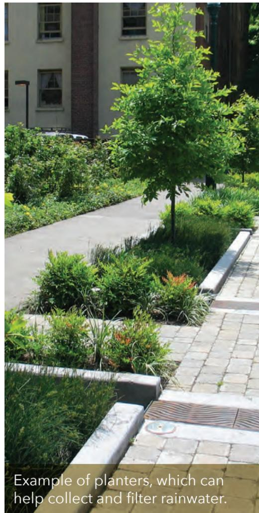
Example of planters, which can help collect and filter rainwater.
