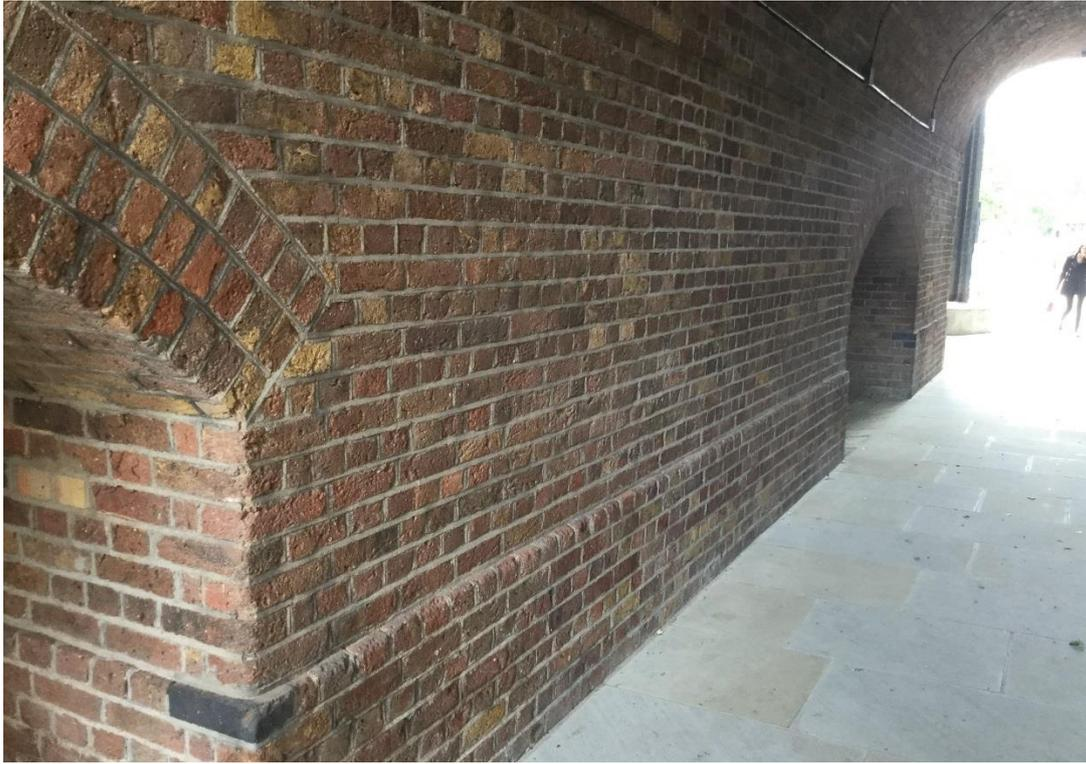
The freshly clean brick work and new paving at Latimer Road Station Bridge
