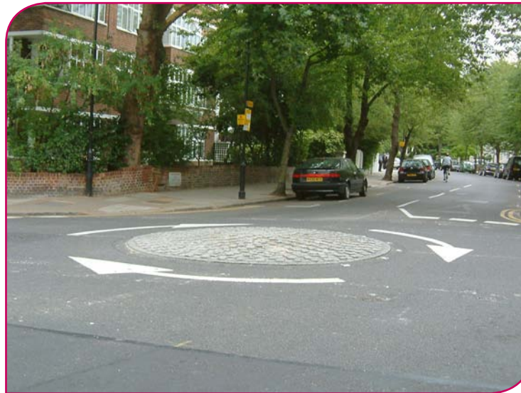
Mini-roundabout with granite setts – Chepstow Villas
