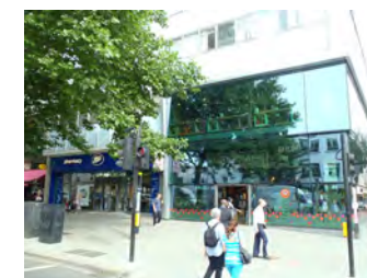
Recent shop front improvements at Notting Hill Gate
