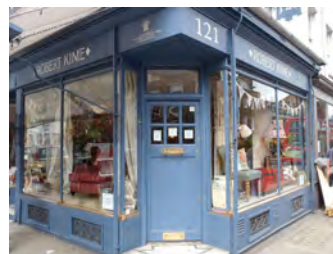
Traditional shop front, Kensington Church Street
