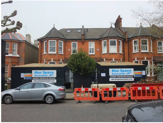
Basement projects in Kelfield Gardens W10, 2014
