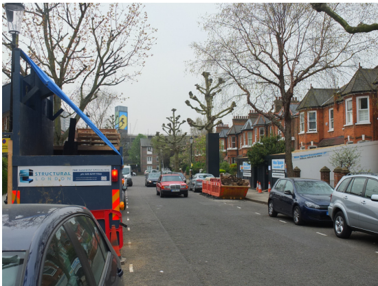
Basement projects in Highlever Road W10, 2014
