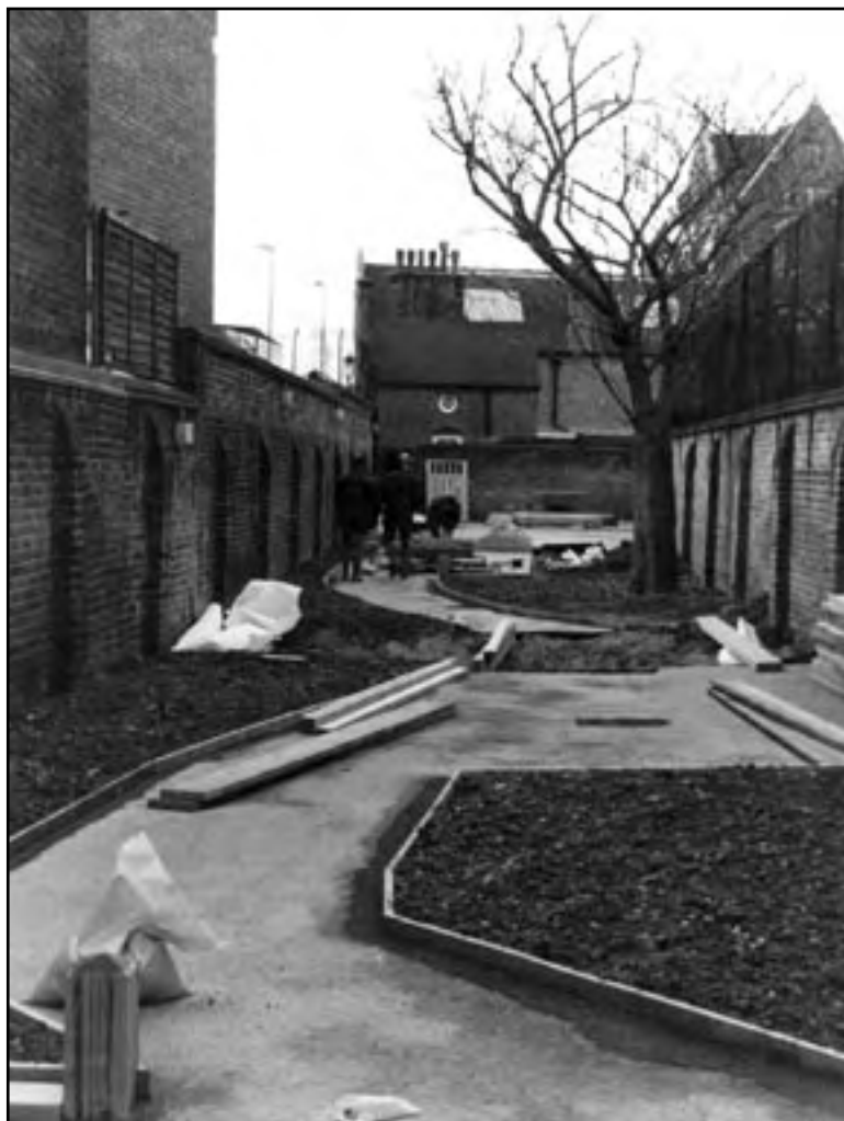
Oxford Gardens Primary School - during construction
