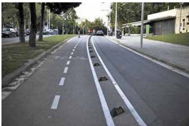
Cycling Exhibit 8: Barcelona example of a low cost Spanish Cycle Track using small bollards bolted to the road, estimated to cost 10%-20% of typical UK cycle tracks [B. Deegan, personal communication] (Photo www.copenhagenize.com ).
