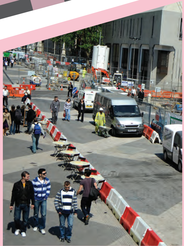
Nearly finished – the works will soon be over
