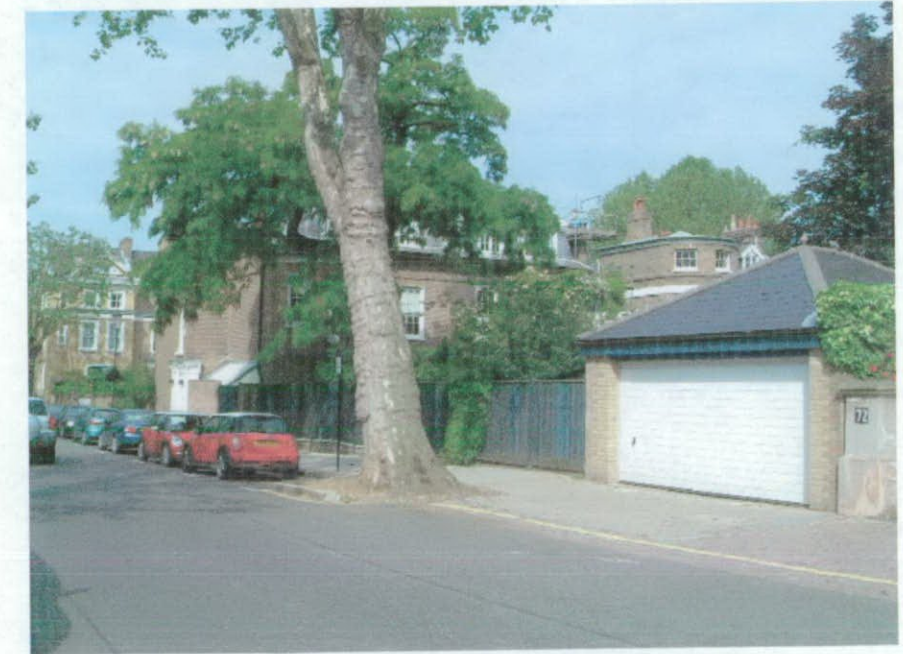
No.2, Garage on Ladbroke Road
