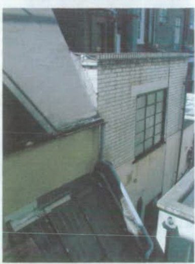
REAR OF No.88
