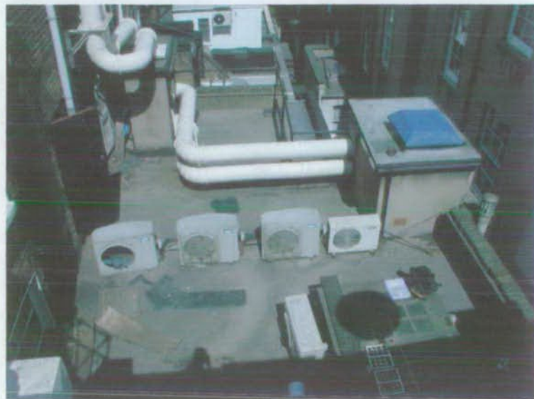
VIEWS DOWN ONTO THE REAR ROOF DECK
