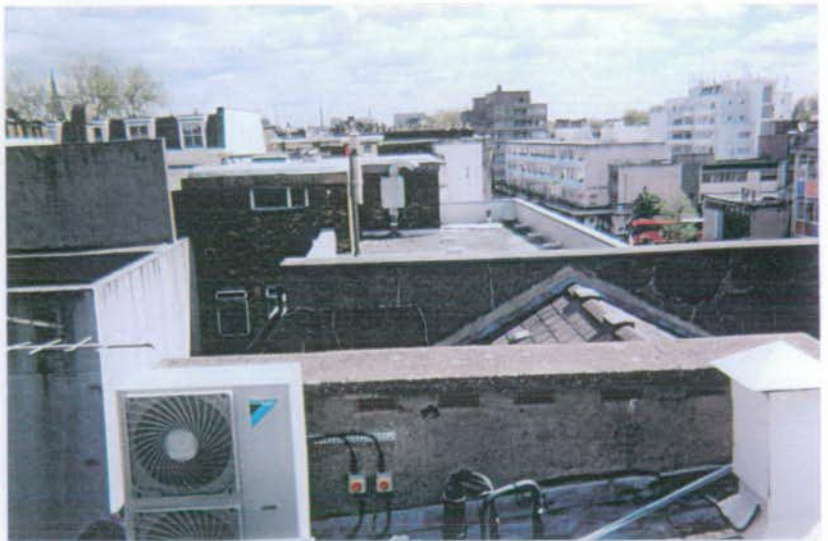
VIEW EAST OVER NO 88
