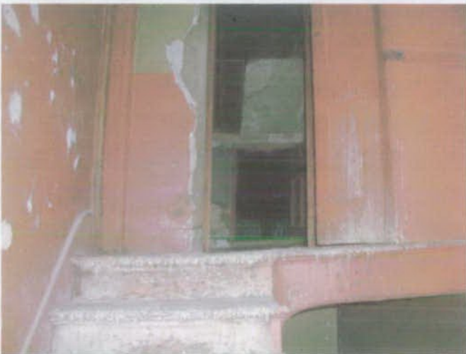
OF ATTIC FLOOR (3 RD )
