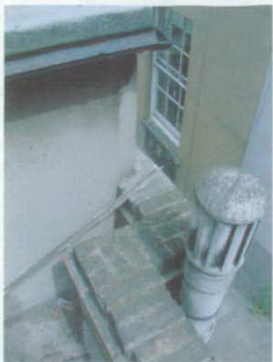
PART OF REAR ROOF OF No.88
