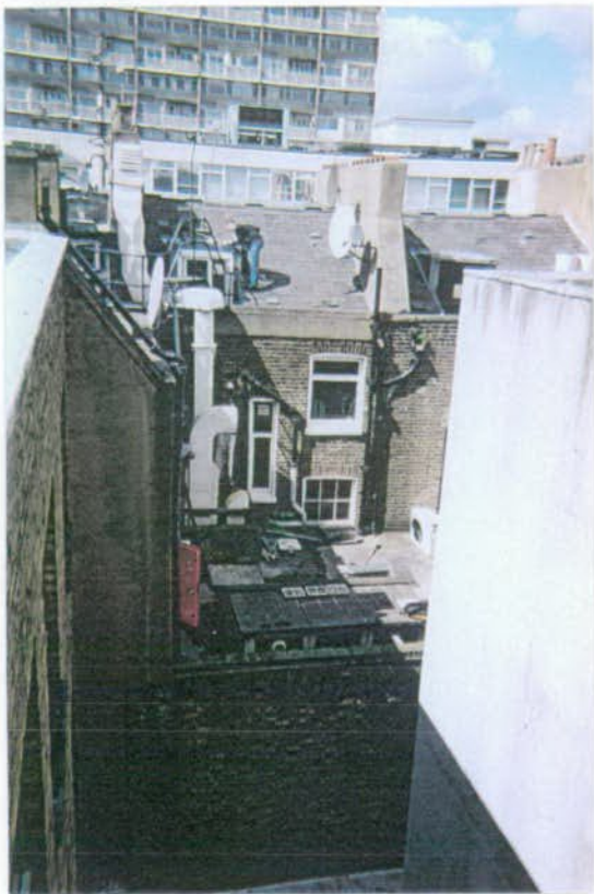
VIEW WEST TO BACK OF N°2
