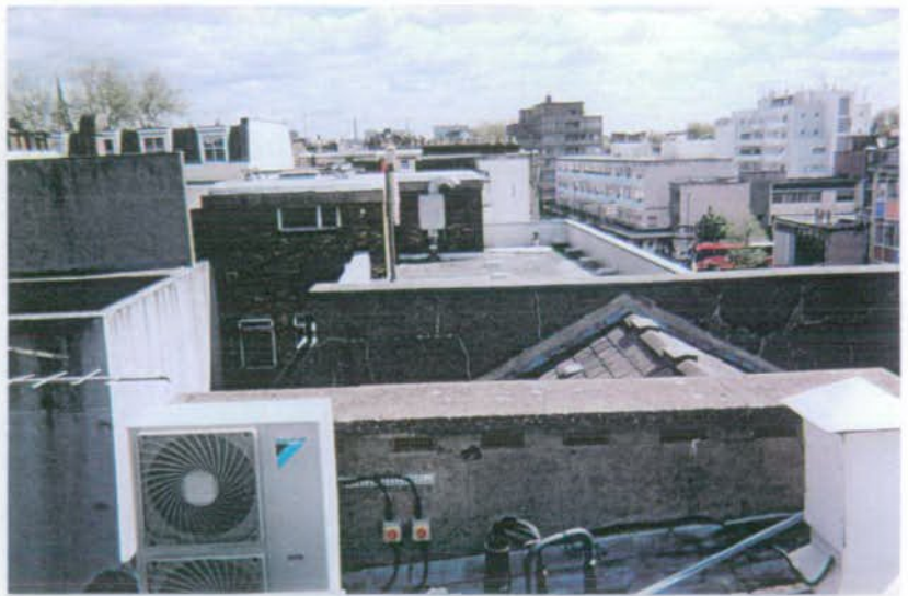
VIEW EAST OVER NO 88
