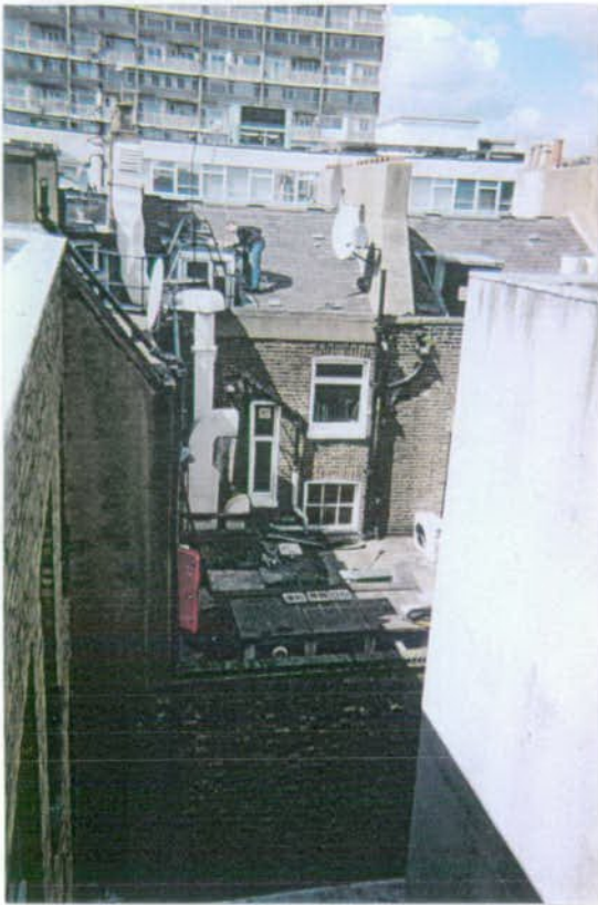
VIEW WEST TO BACK OF N°2
