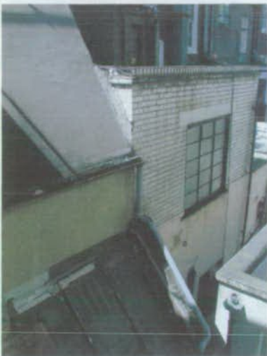
REAR OF No.88
