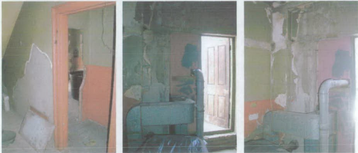
VIEWS OF SECOND FLOOR OF No.4
