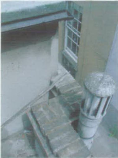
PART OF REAR ROOF OF No.88
