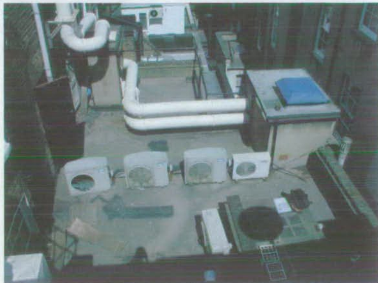
VIEWS DOWN ONTO THE REAR ROOF DECK
