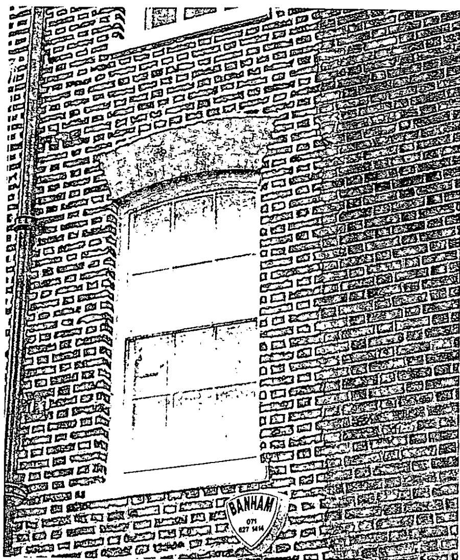
Poor repointing can cause irreversible damage to a building and ruin its appearance
