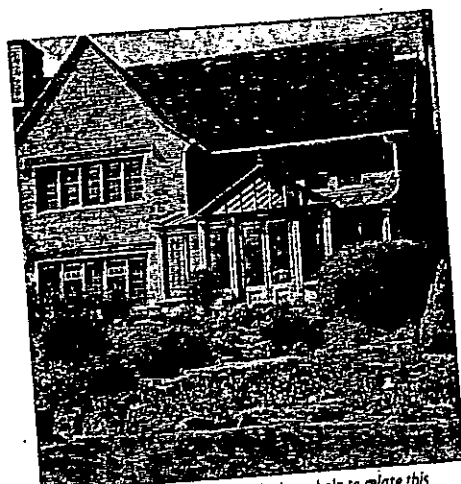
Leaded lights set in green painted joinery help to relate this conservatory to the original 1930s architecture of the house and its garden. (Vale Garden Houses)
