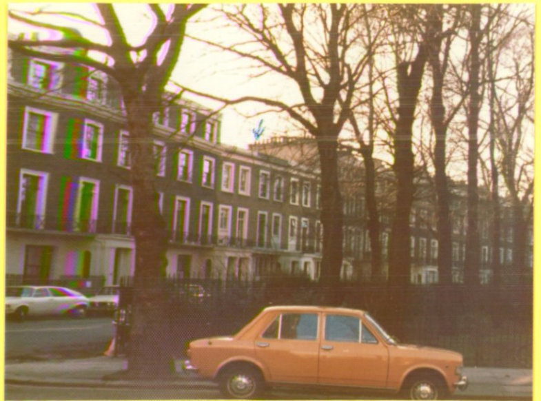
VIEW OF HOUSE FROM THE NORTH EAST
