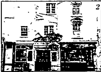
1 Category B shopfronts in the Lancer Square development
