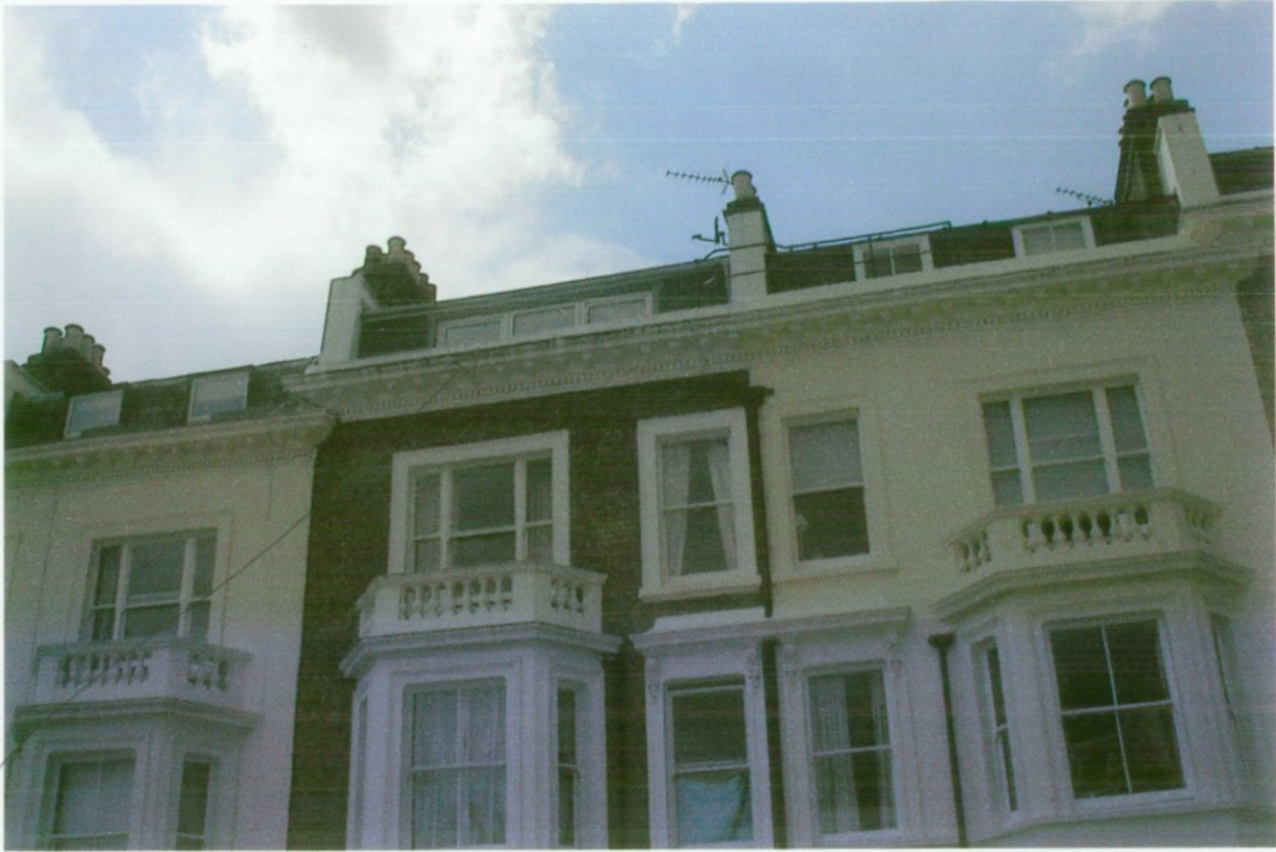
Existing Dormer windows
