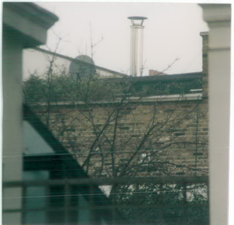
4 - DETAIL OF EXISTING TERRACE
