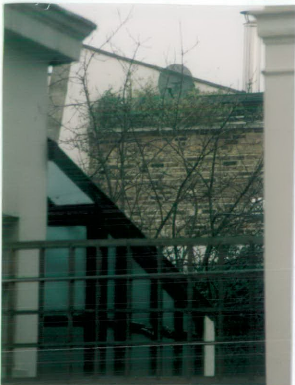
3 - DETAIL OF EXISTING TERRACE
