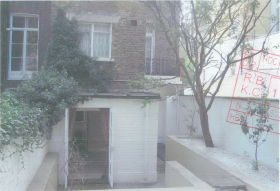
View of rear of Basement at 28 Fawcett Street
