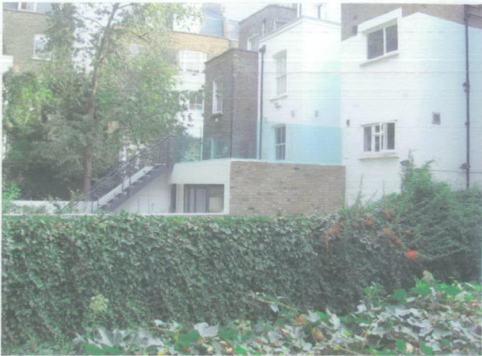
View of extension to property 2 houses away
