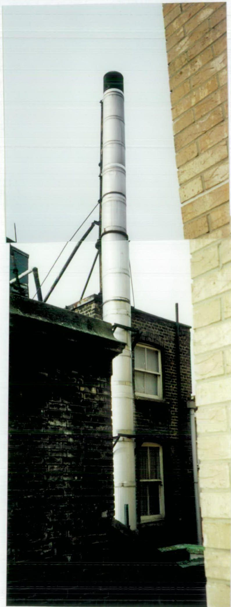
Photo 17. Existing rear elevation of 1, De Vere Gardens, detail
