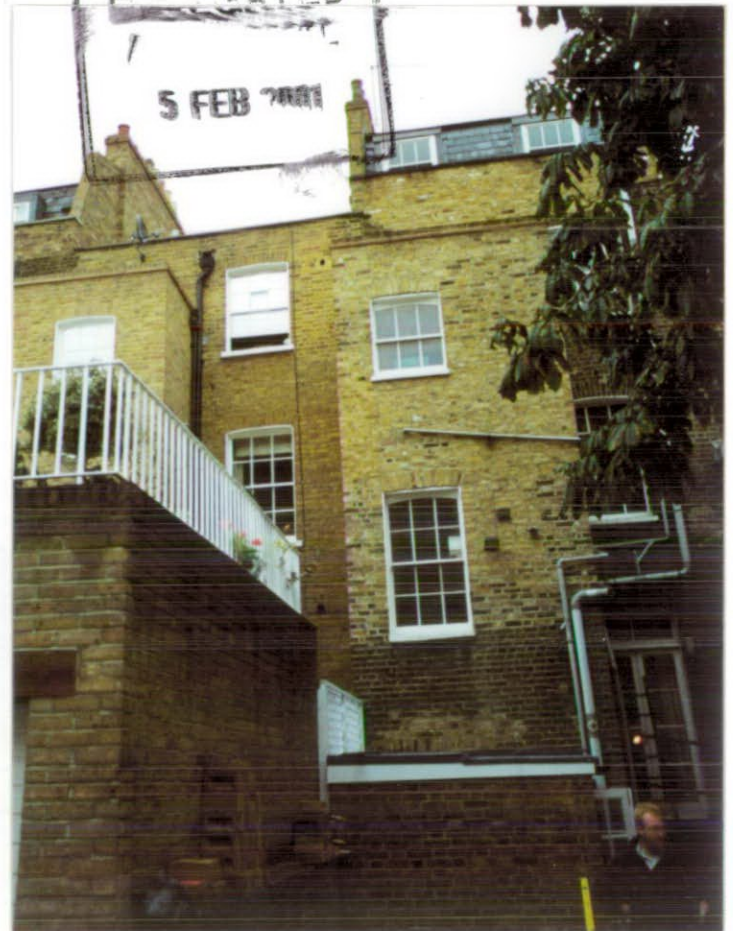
REAR RENOVATION IN NEIGHBOUR
