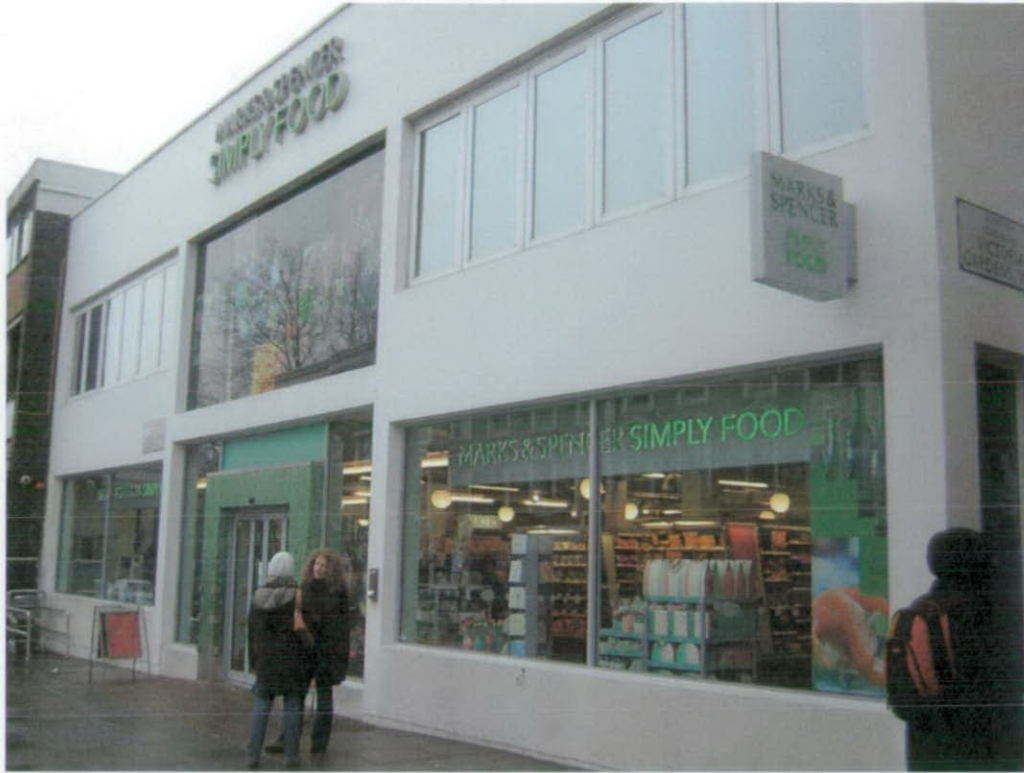
9. Marks and Spencer's located to the west of the proposal site
