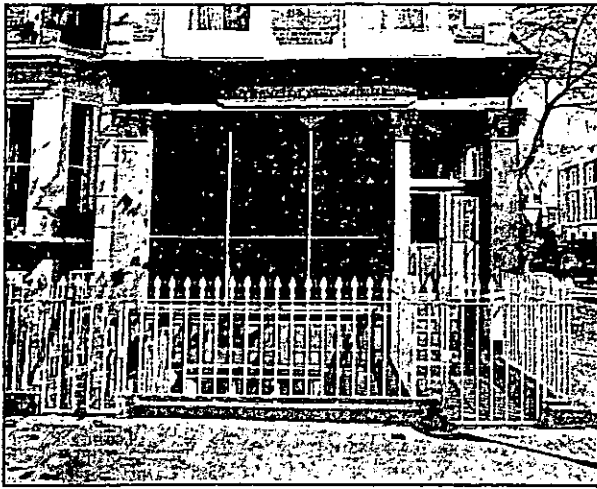
11 31 Abingdon Road. A finely detailed corner shop in a predominantly residential area. This is a typical example of the use of pilasters to support the cornice, without corbel brackets.
