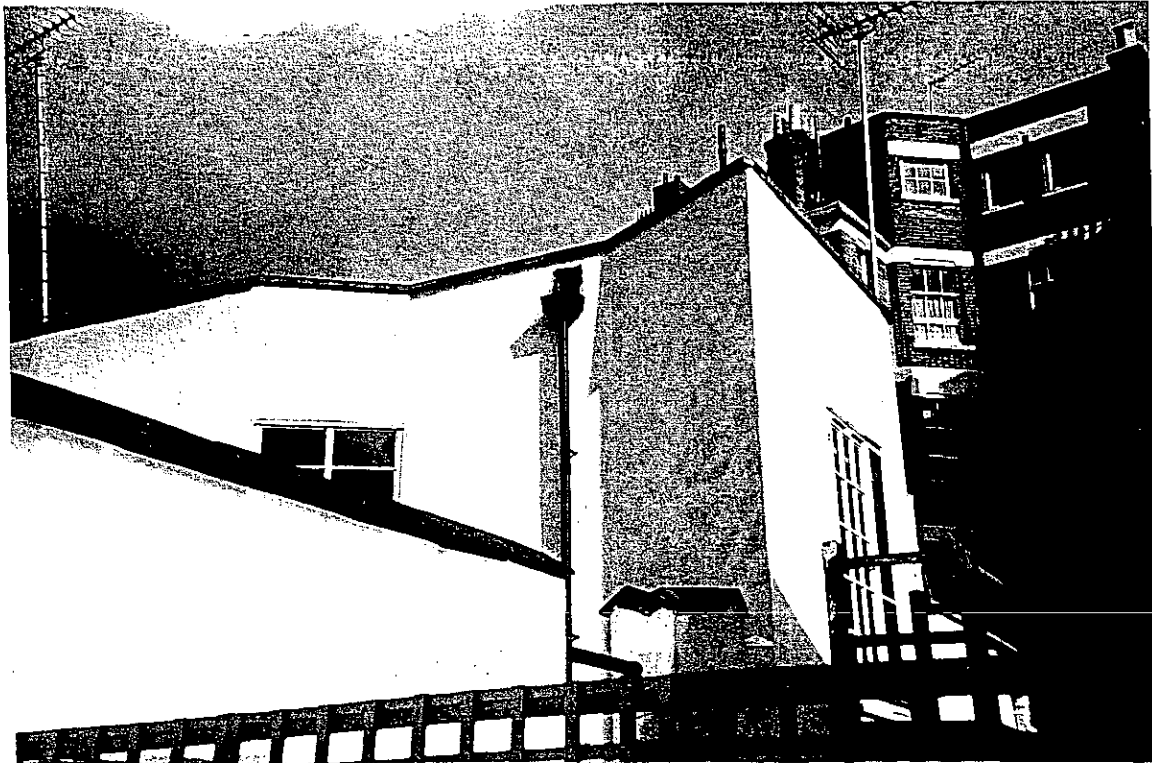
VIEW OF EXTENSION AT 2ND FL LEVEL TO NO 20 TAKEN FROM REAR 1ST FL TERRACE OF NO 18.
