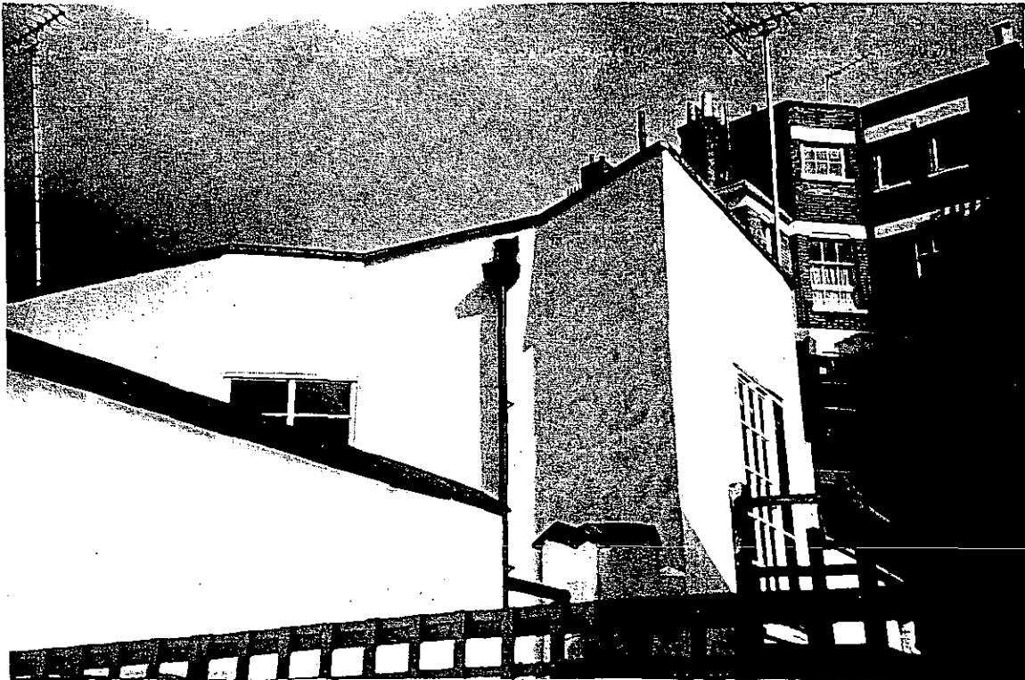
VIEW OF EXTENSION AT 2ND FL LEVEL TO NO 20 TAKEN FROM 1ST FL TERRACE OF NO 15.
