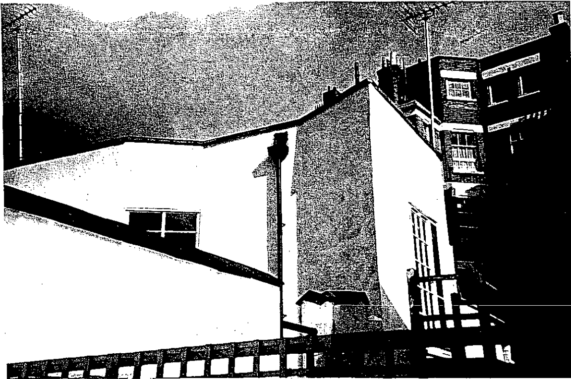
VIEW OF EXTENSION AT 2ND FL LEVEL TO NO 20 TAKEN FROM REAR 1ST FL TERRACE OF NO 18.
