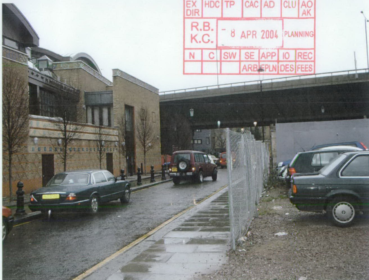
ST ERVANS ROAD . LONDON W10 - EXISTING VIEWS
