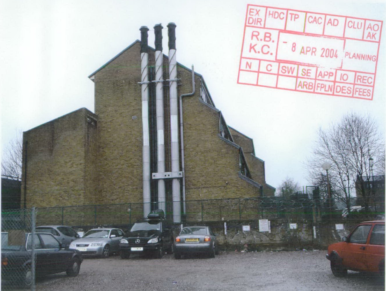
ST ERVANS ROAD . LONDON W10 - EXISTING VIEWS
