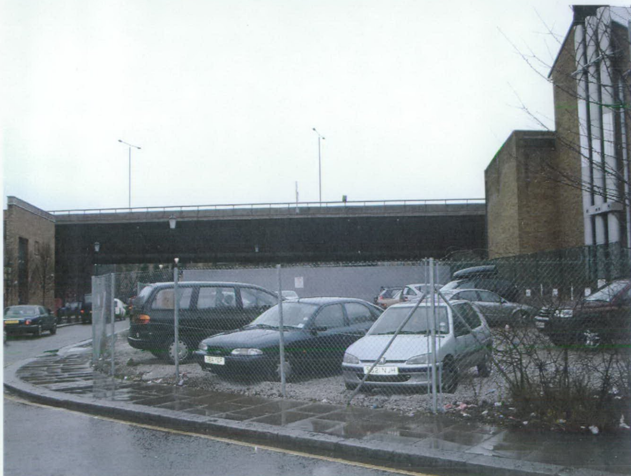
ST ERVANS ROAD . LONDON W10 - EXISTING VIEWS
