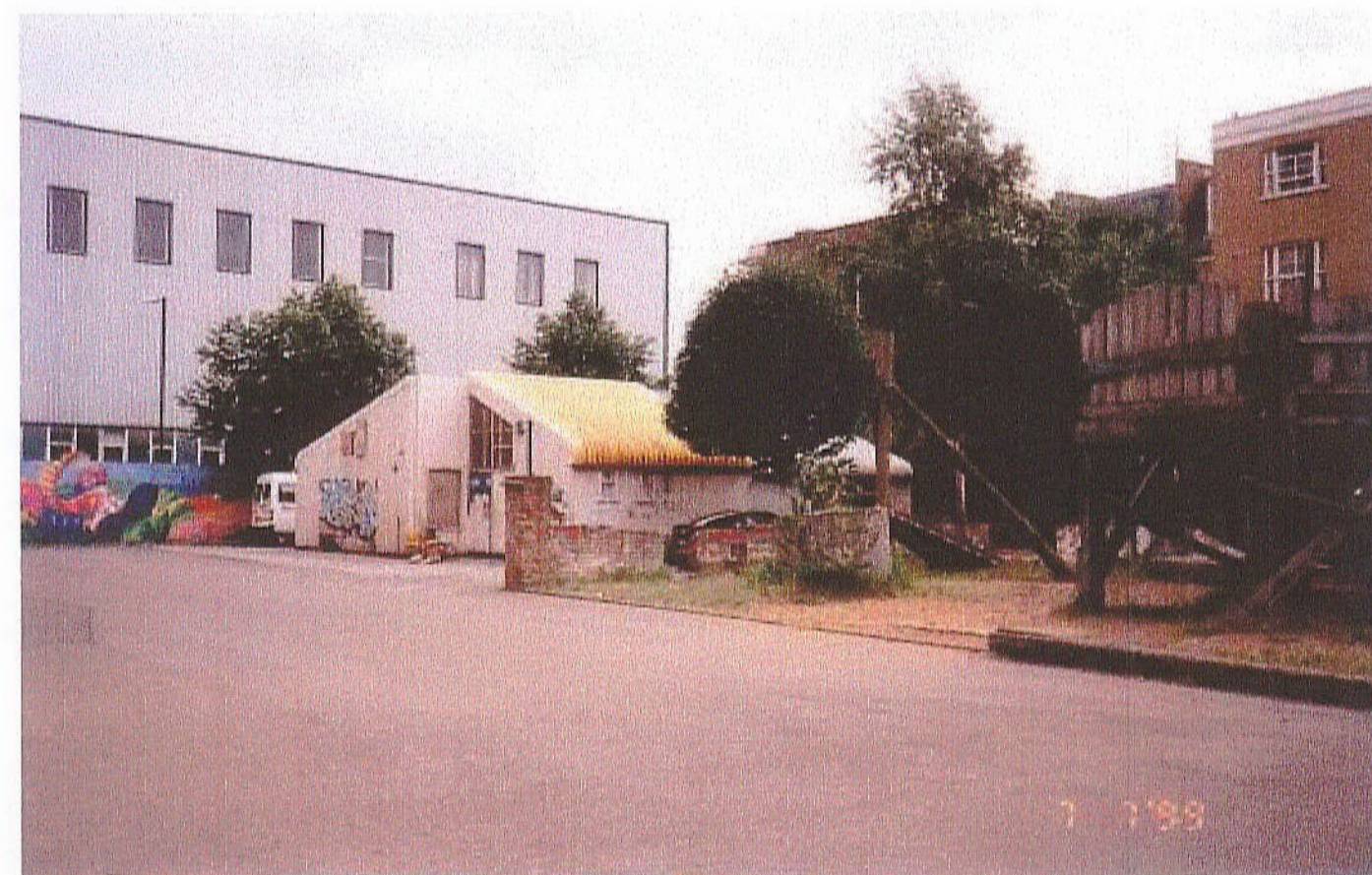
Existing building viewed from North East
