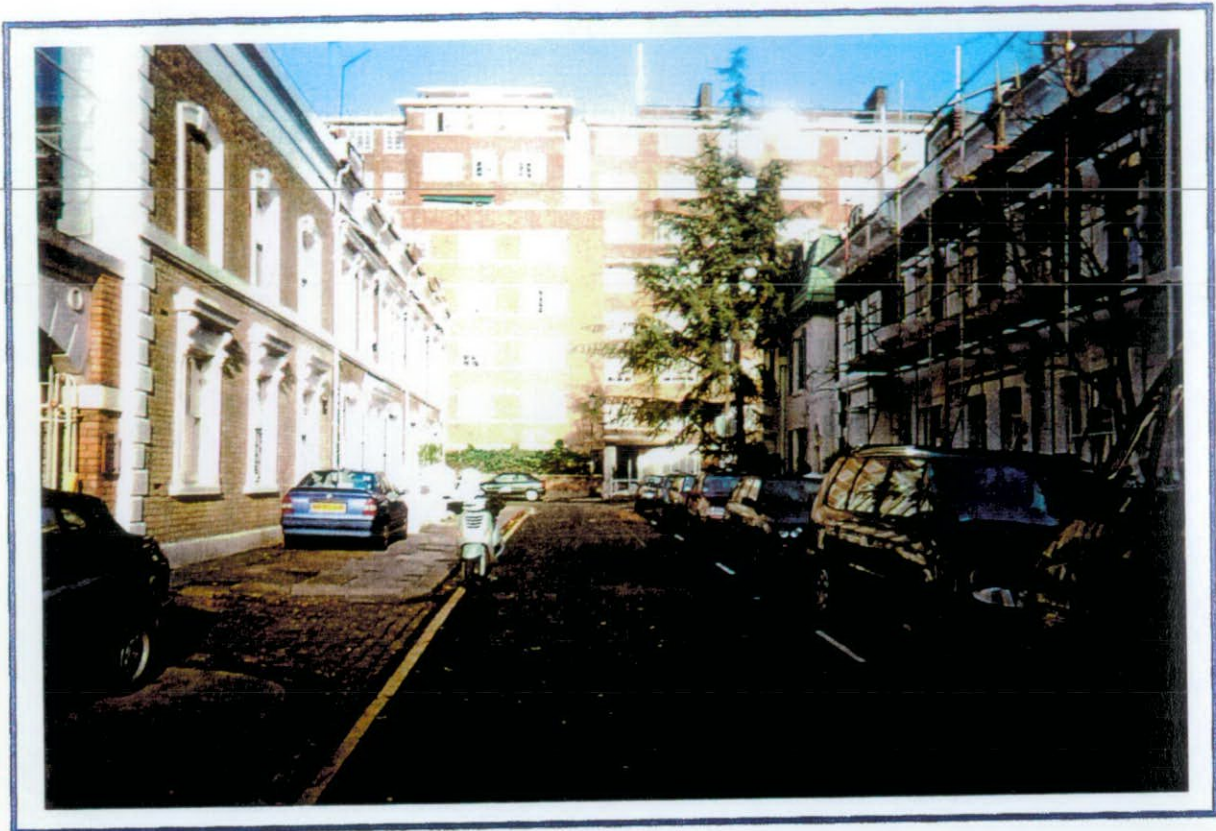
KELSO PLACE – LOOKING NORTH
