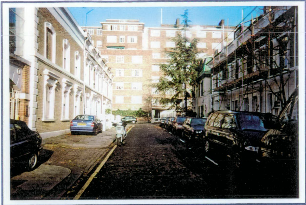
KELSO PLACE – LOOKING NORTH
