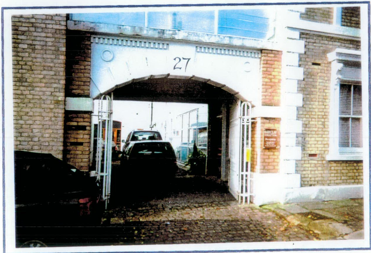
PAVEMENT CROSSOVER & GROUND FLOOR ENTRANCE
