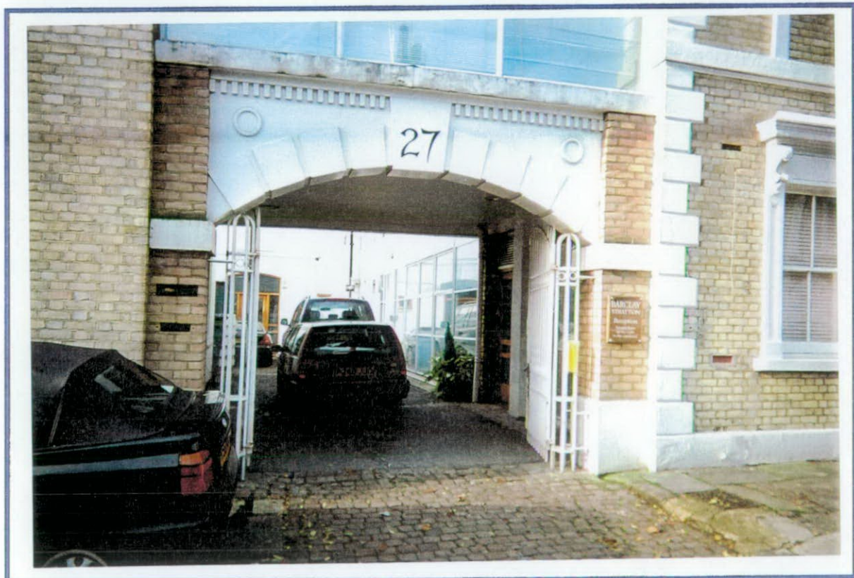
PAVEMENT CROSSOVER & GROUND FLOOR ENTRANCE
