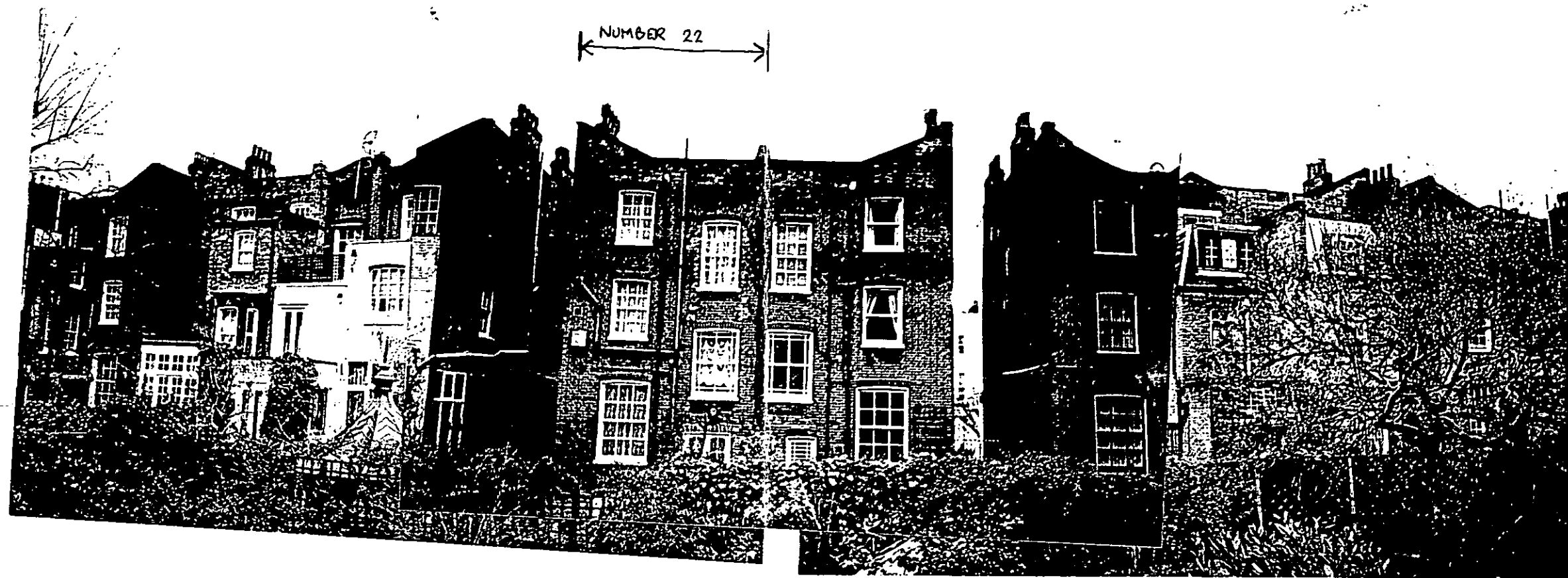
REAR OF NUMBER 22 WITH ADJACENT BUILDINGS
