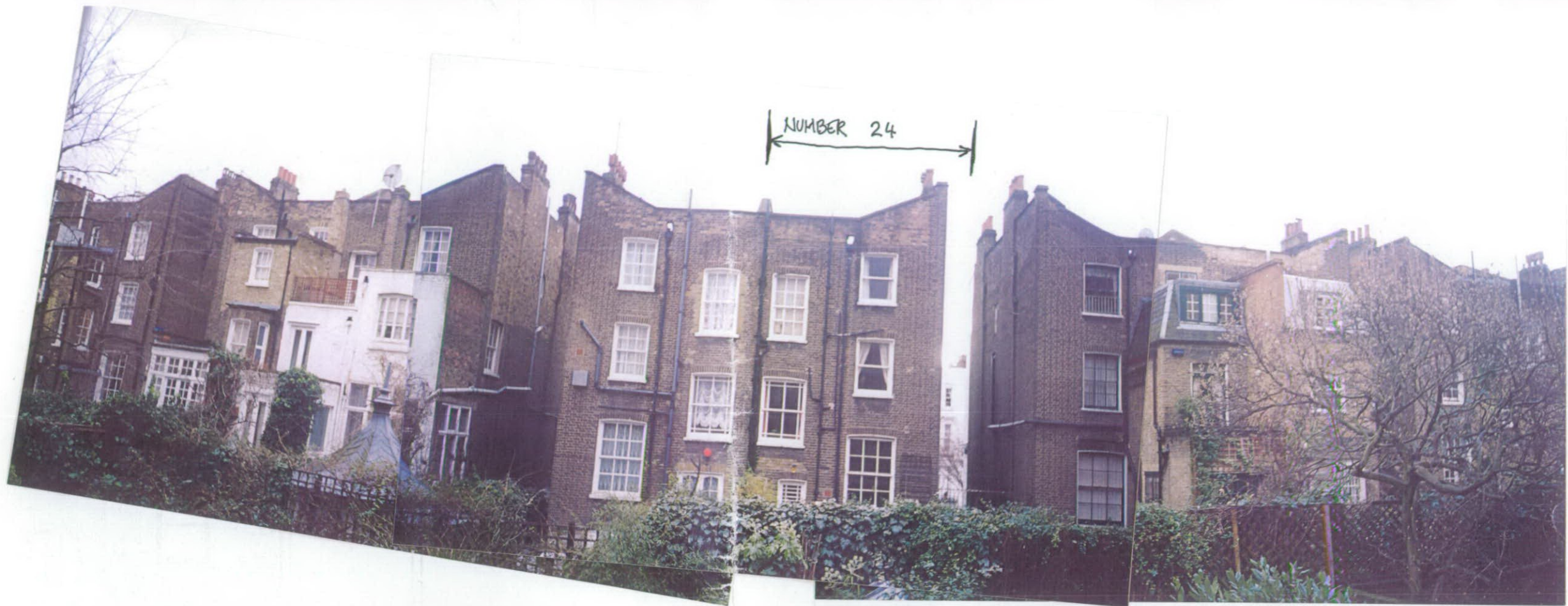
REAR OF NUMBER 24 WITH ADJACENT BUILDINGS
