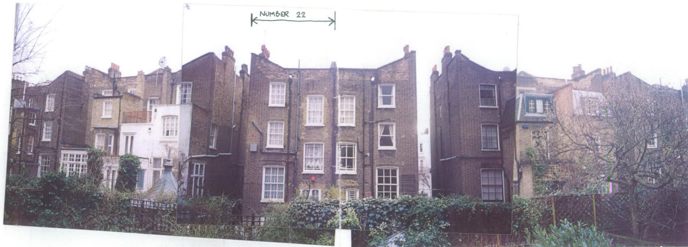
REAR OF NUMBER 22 WITH ADJACENT BUILDINGS
