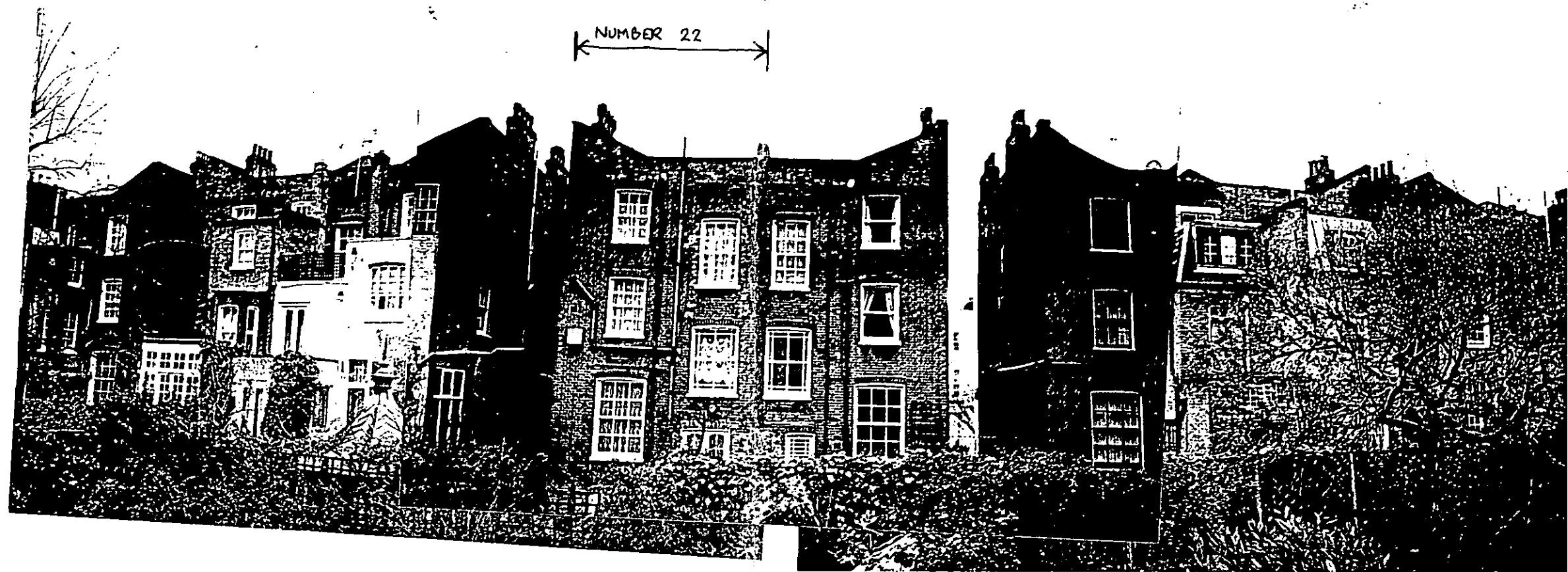
REAR OF NUMBER 22 WITH ADJACENT BUILDINGS
