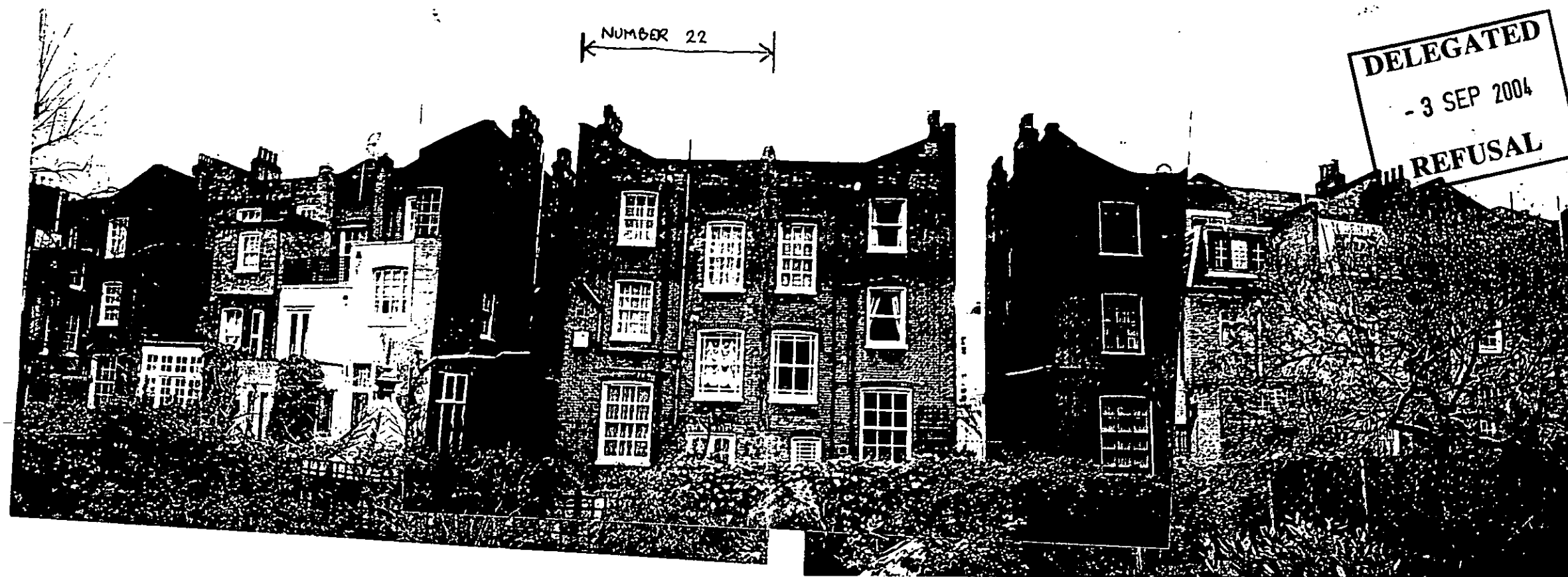
REAR OF NUMBER 22 WITH ADJACENT BUILDINGS
