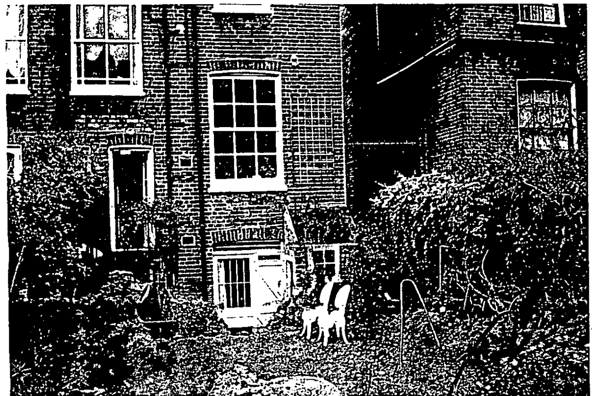
REAR OF NUMBER 24 AT GARDEN LEVEL
