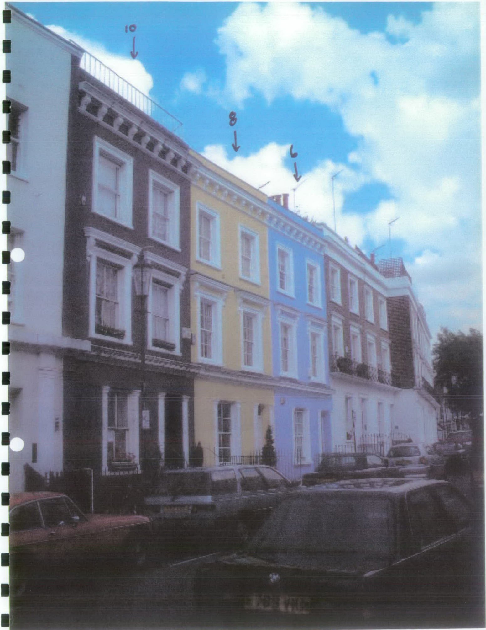
Front elevation of 6, 8, 10 Penzance Place.
