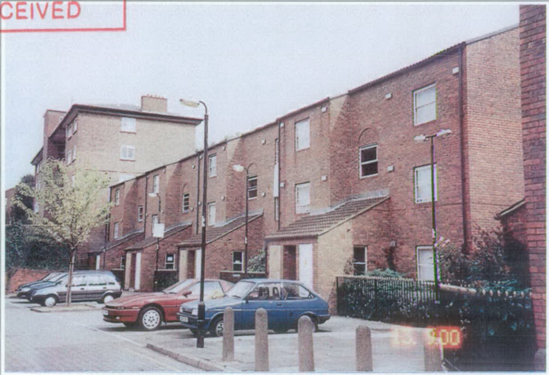
Rear elevation of flat 13 to 36
