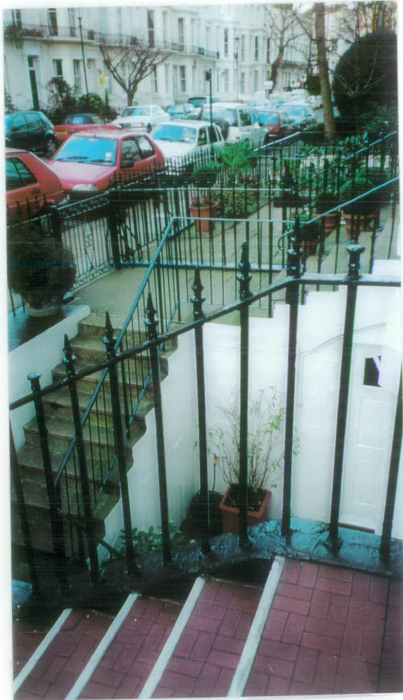
FRONT LIGHT-WELL TO ADJACENT PROPERTY, No. 24 CAMPDEN GROVE.
