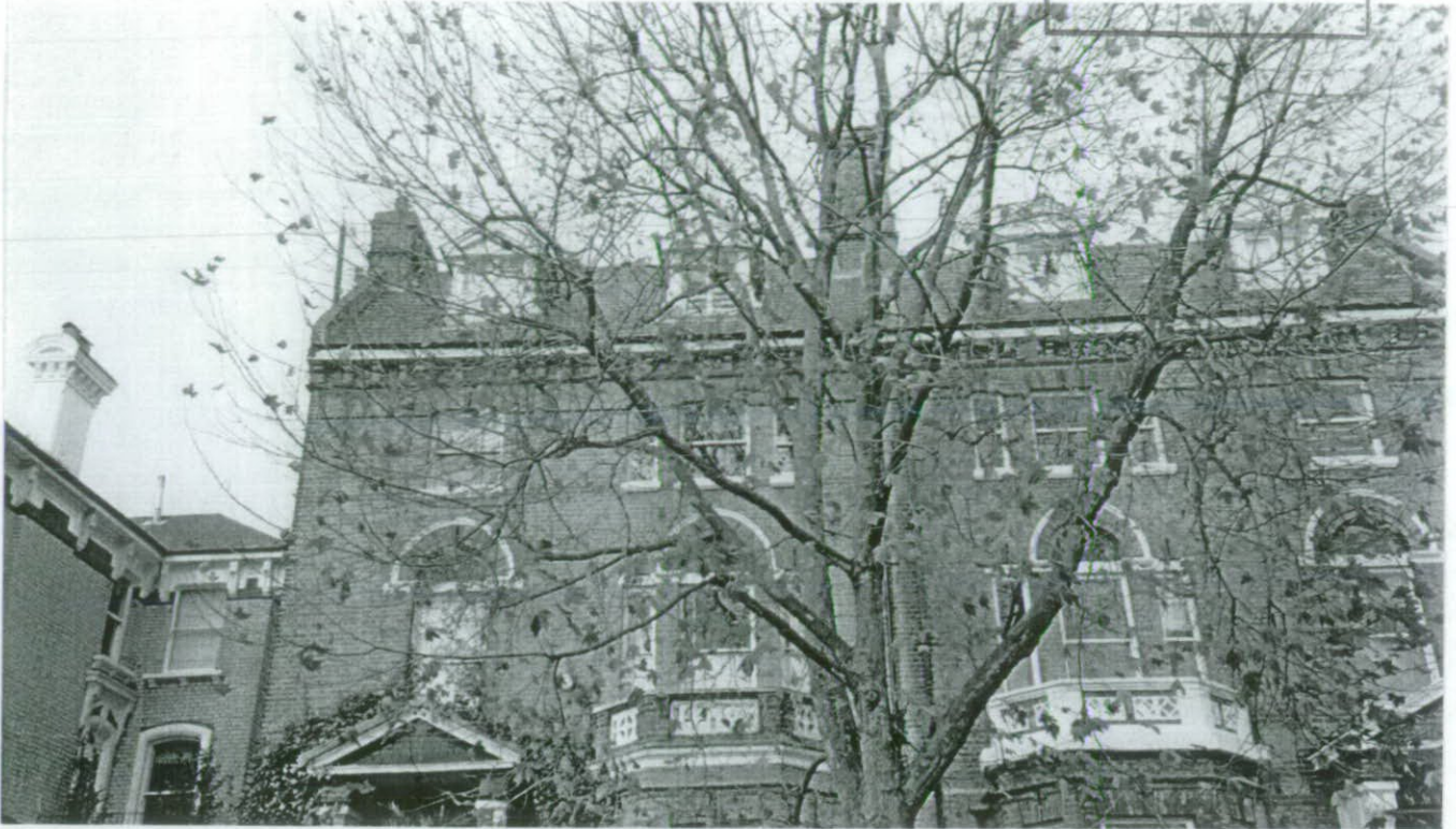
Front view of the house to the left and an adjoining house (20 Tregunter Road)
