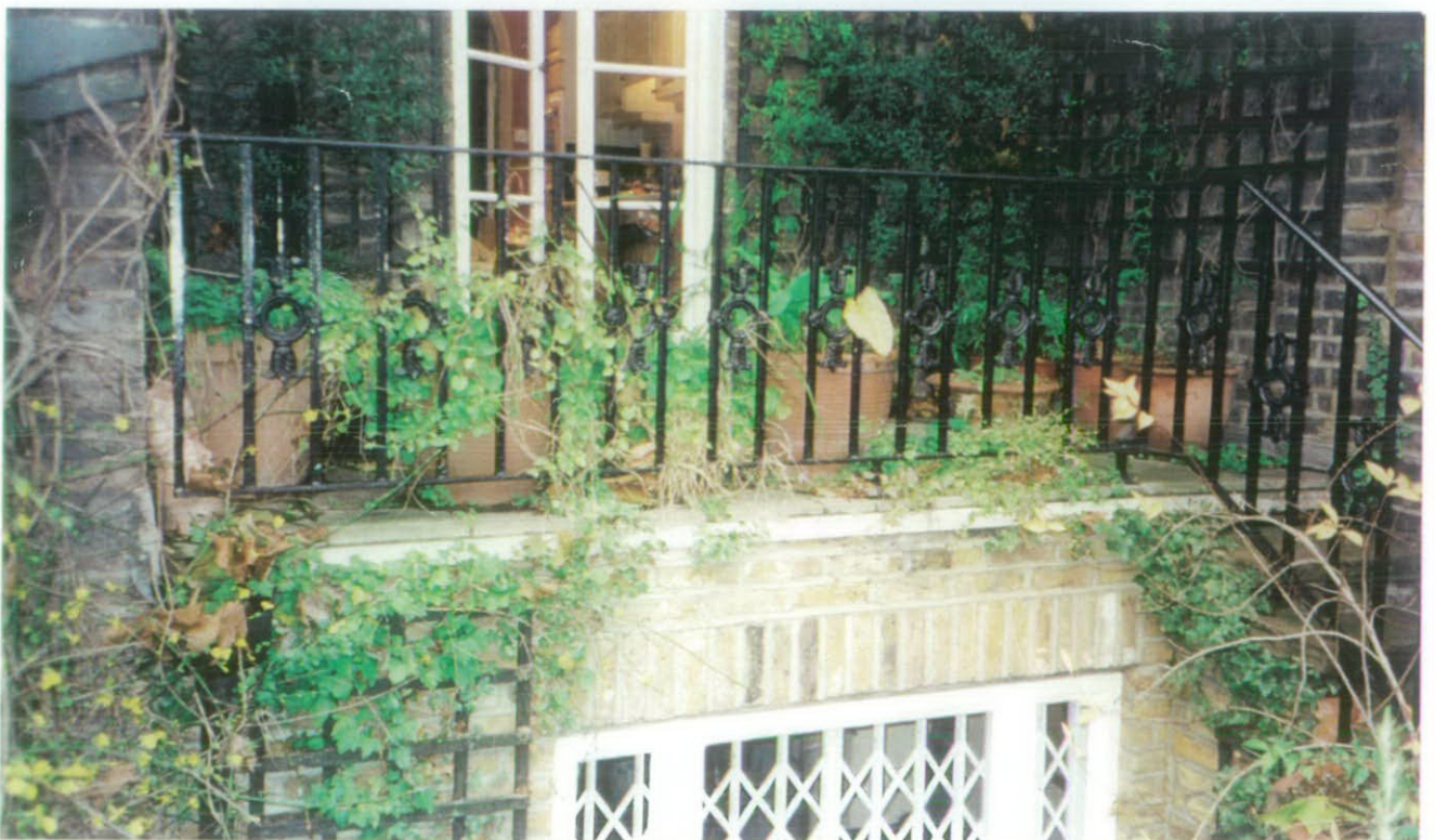
PO2 View of existing balustrade
