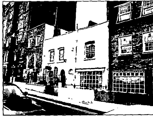
Oversized dormers in Peel Street (far left)
