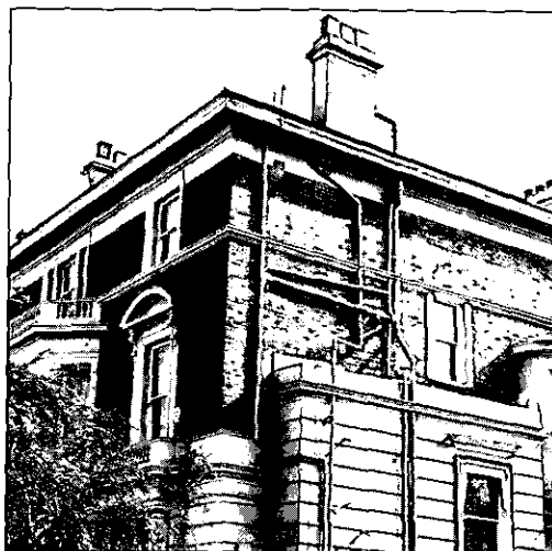
Excessive pipework on walls, roofs and around decorative detail (left)
