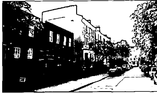
Listed terraces in Stafford Terrace frame a glimpse of St Mary Abbot's spire (far left)
