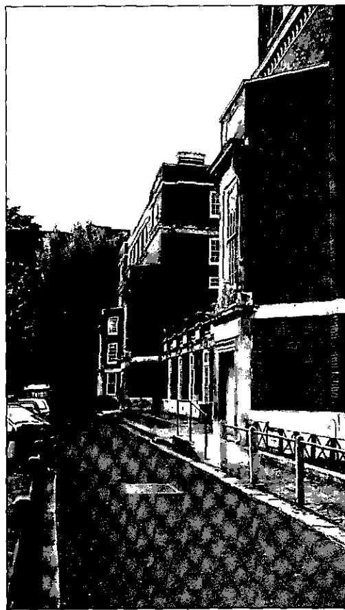
C1. Works frontage, Jameson Street (far left)
