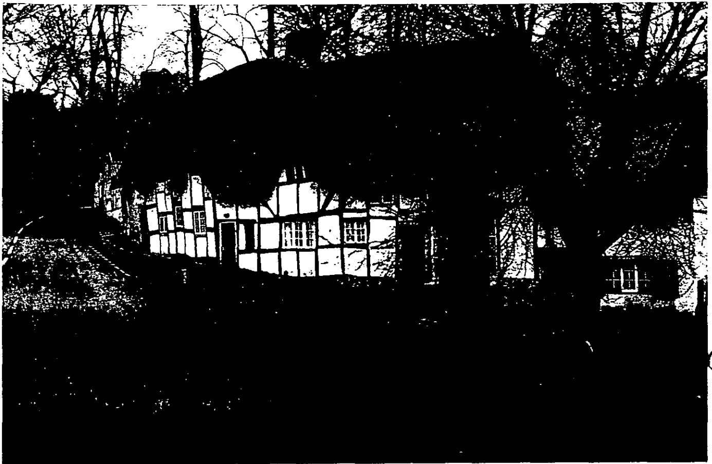
Wherwell, Hants Vernacular building traditions like timber frame construction or thatching techniques should be studied and recorded. (Geoff Noble)
