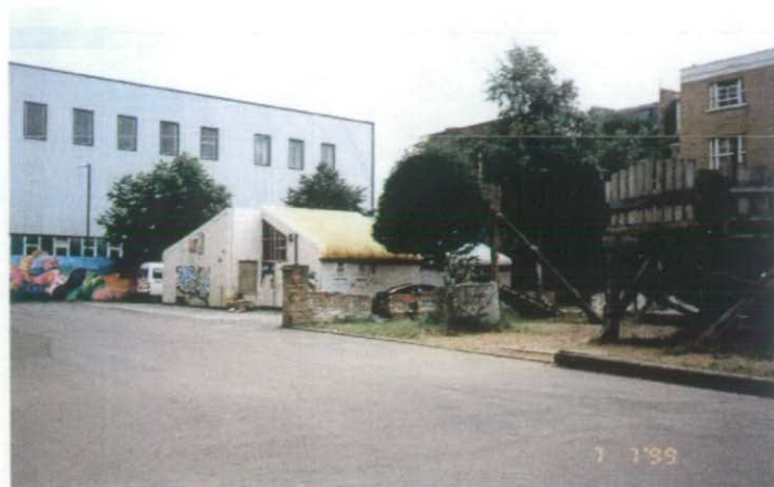
Existing building viewed from North East
