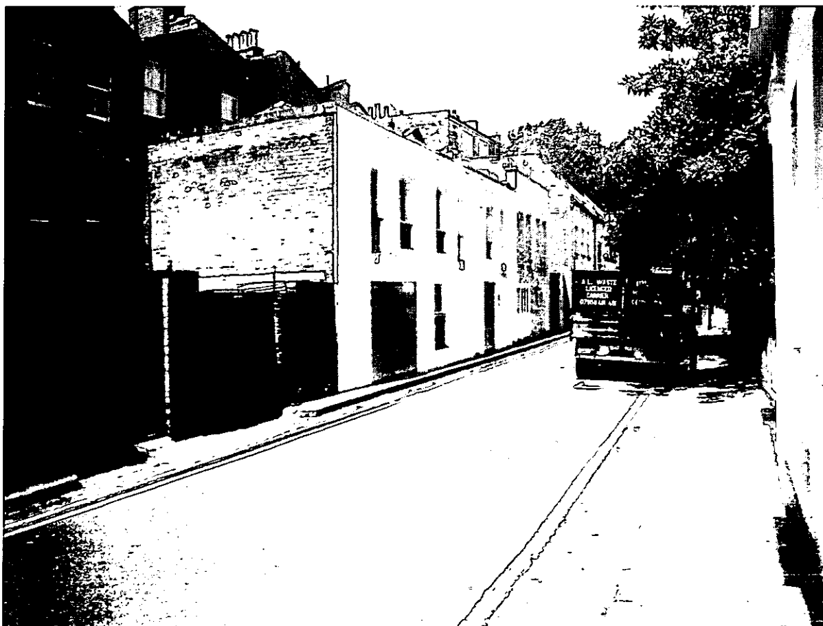
View of property after works
