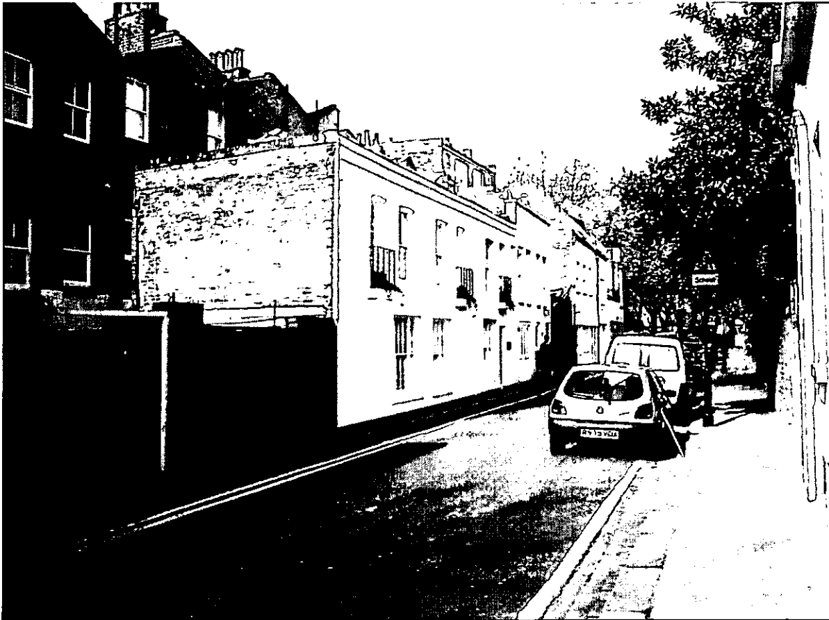
View of property before works
