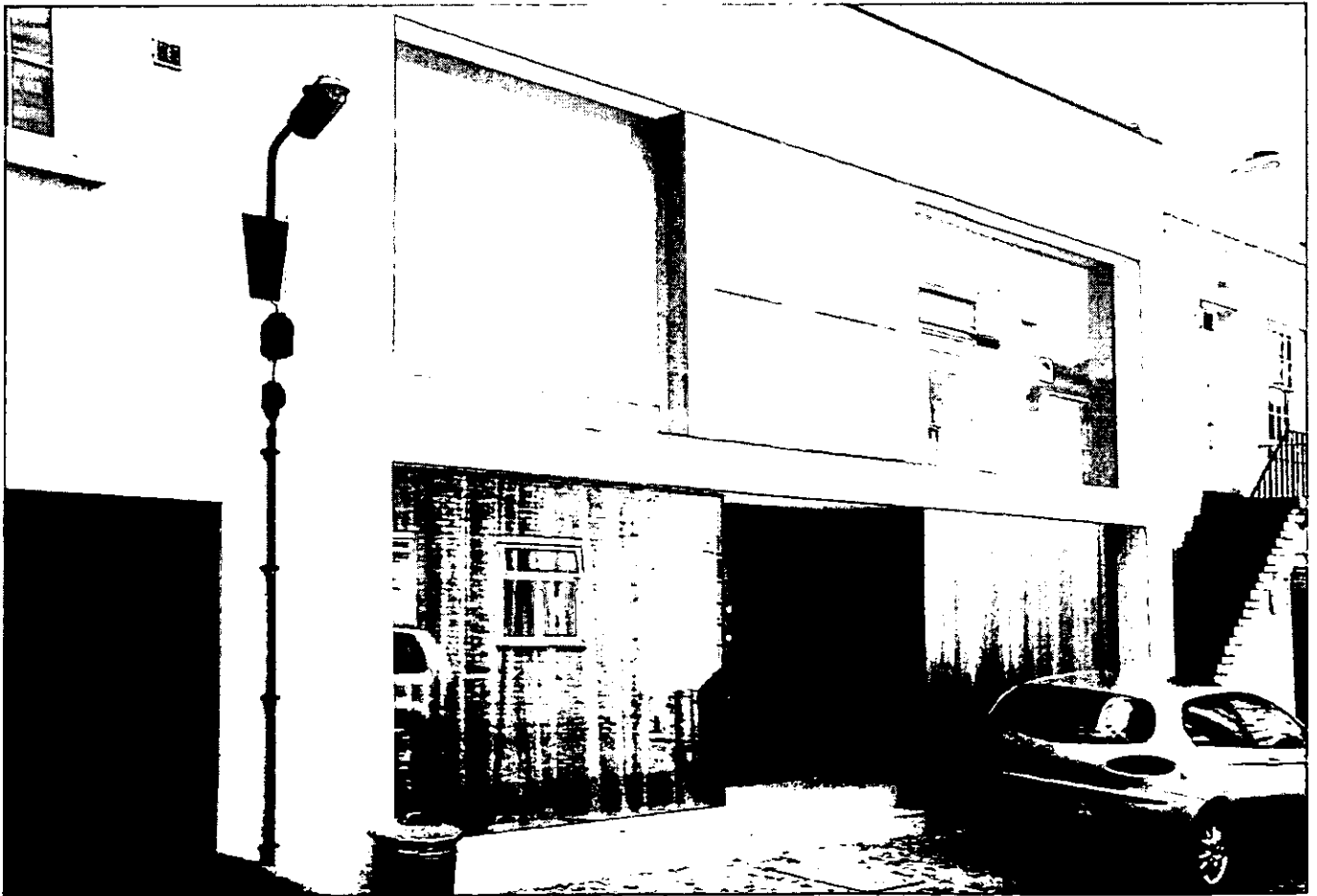
View 16. 13 Norland Place, in the proximity of Pottery Lane
